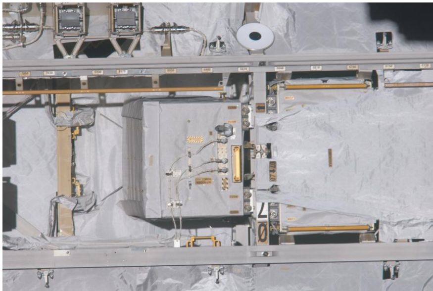
Figure 2. Close up view of the Loop A Pump Module worksite on the front face of the S1 truss segment. NASA image s134e010540.
