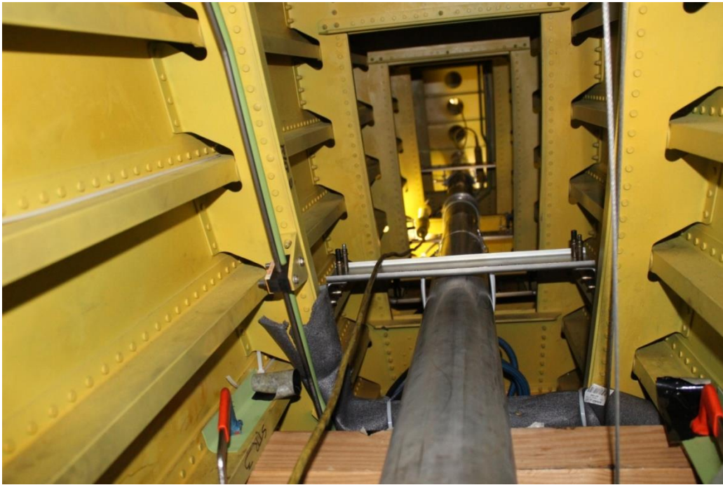
Figure 8: Duct installation inside the vertical fin
