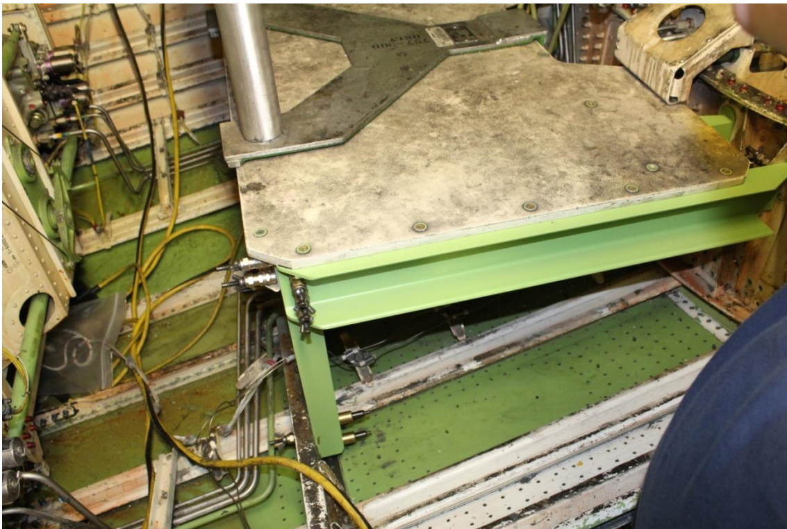
Figure 15: Structural stiffeners under the maintenance platform
