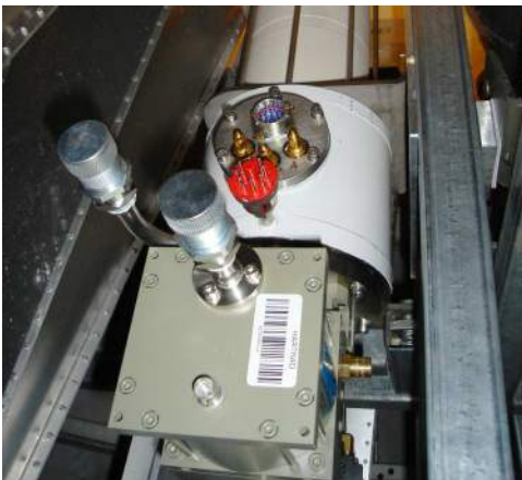
Fig. 4 The 22 GHz receiver, installed on the 26 m on 23 April 2014.
