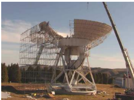
Fig. 1 The dismantling of the 25-m dish in April.
