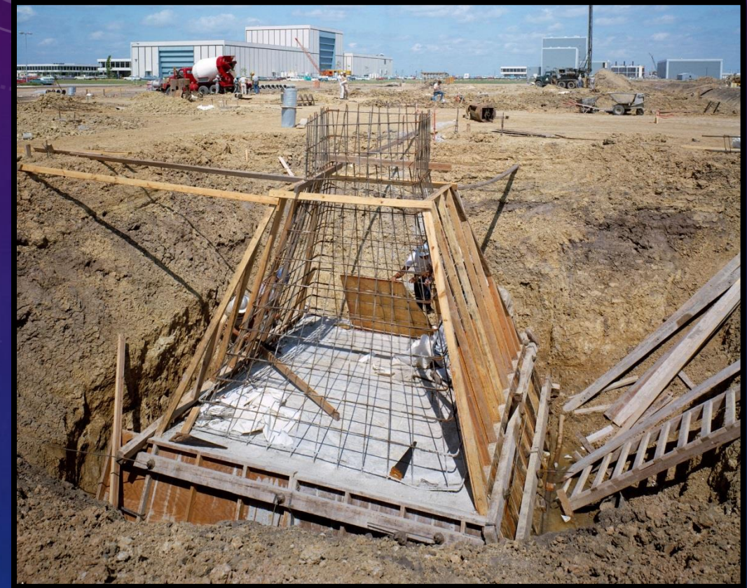
Bldg. 31 Foundation Poured in 1965 (Bldg. 10 in background)
