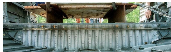
(d) Close-up rear view of the installed conusoid
