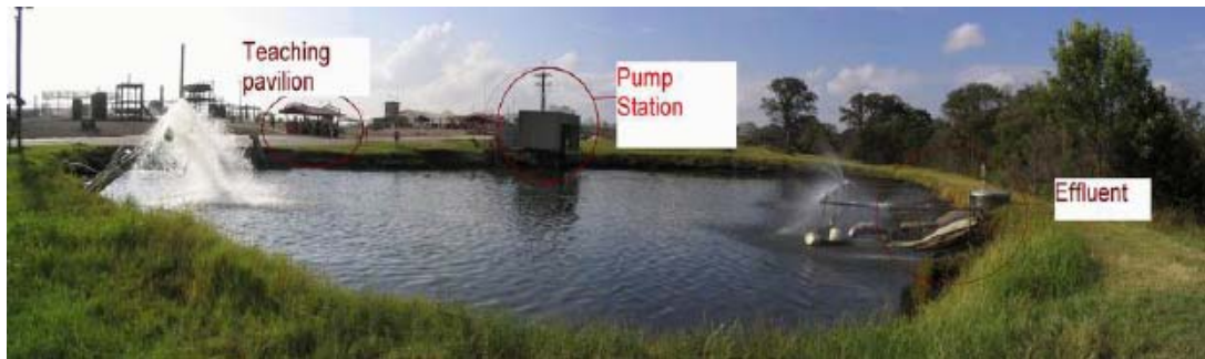
Figure 9. View of Outfall Tank
