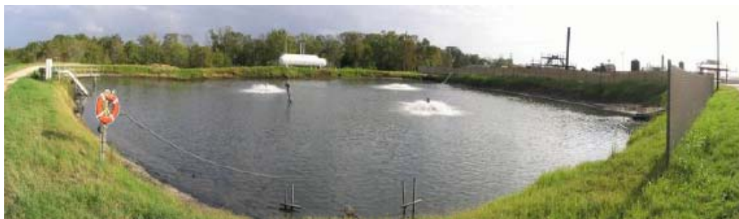
Figure 8. View of the Aeration Tank
