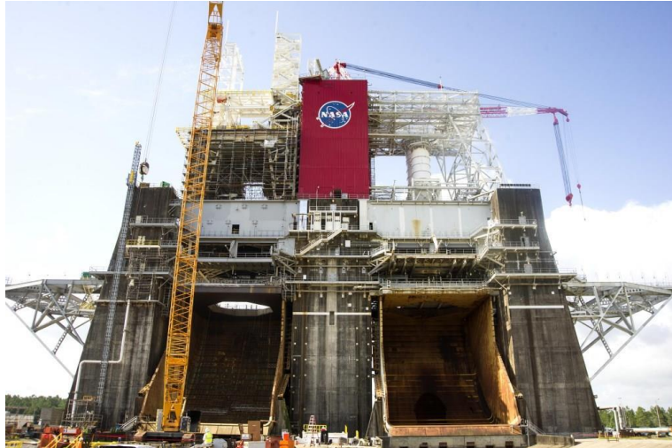
Figure. X: Structural steel for core stage testing erected on B-2 test stand at SSC site.
