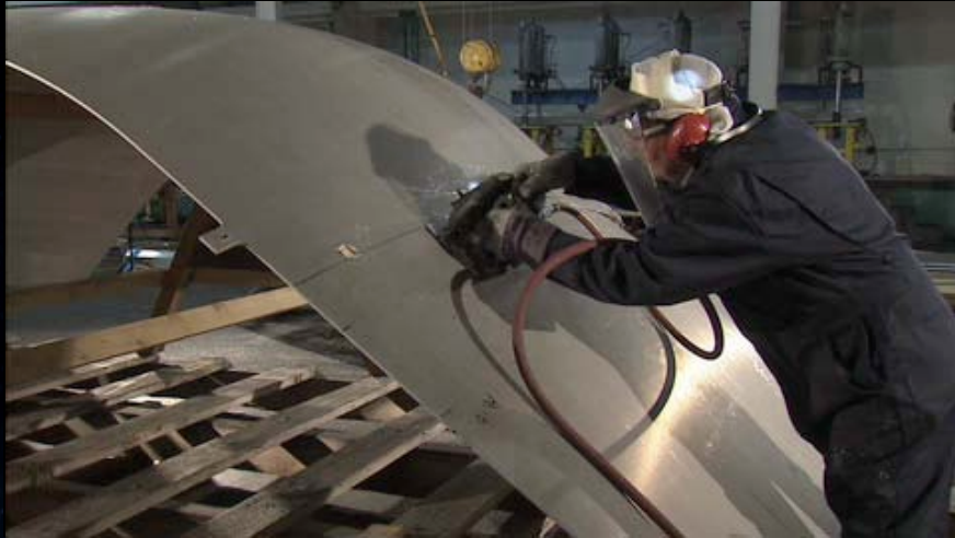
Dome Gore Panel Fabrication Los Angeles, CA
