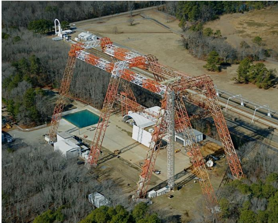
Figure 1 - Landing and Impact Research Facility (LandIR)
