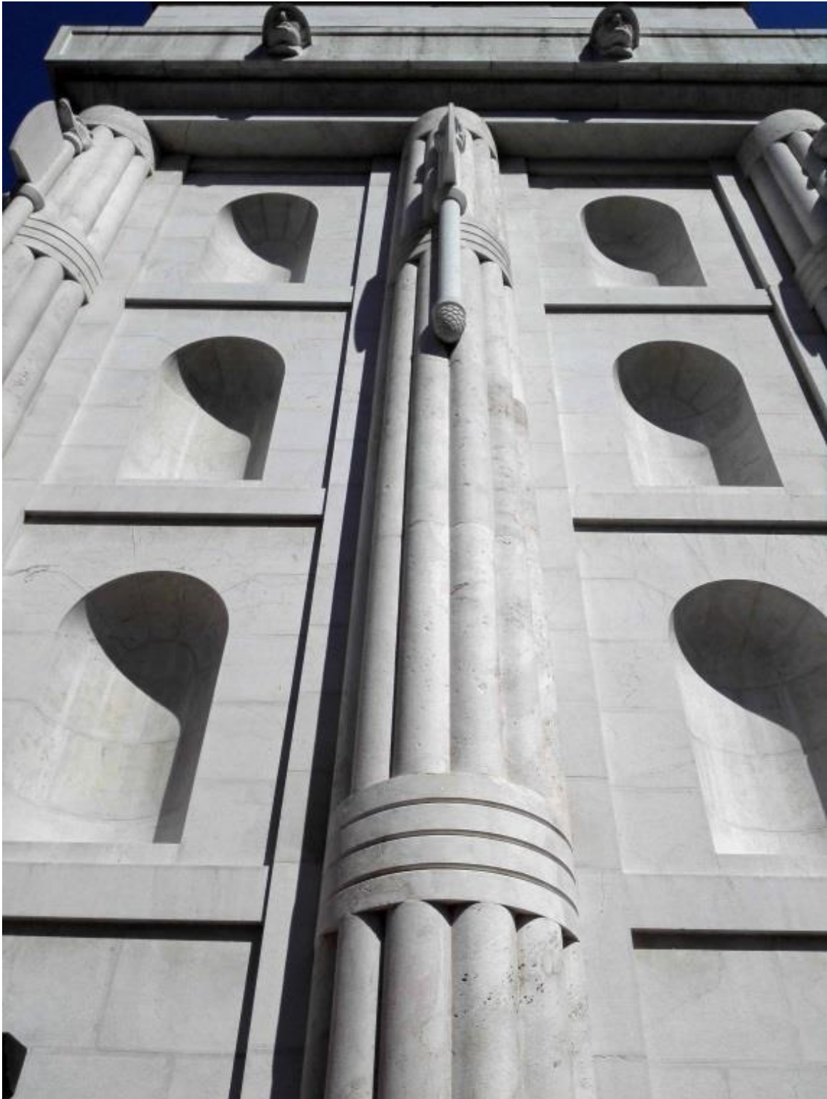
Figure 25 Romanesque-arched niches on the external facade
