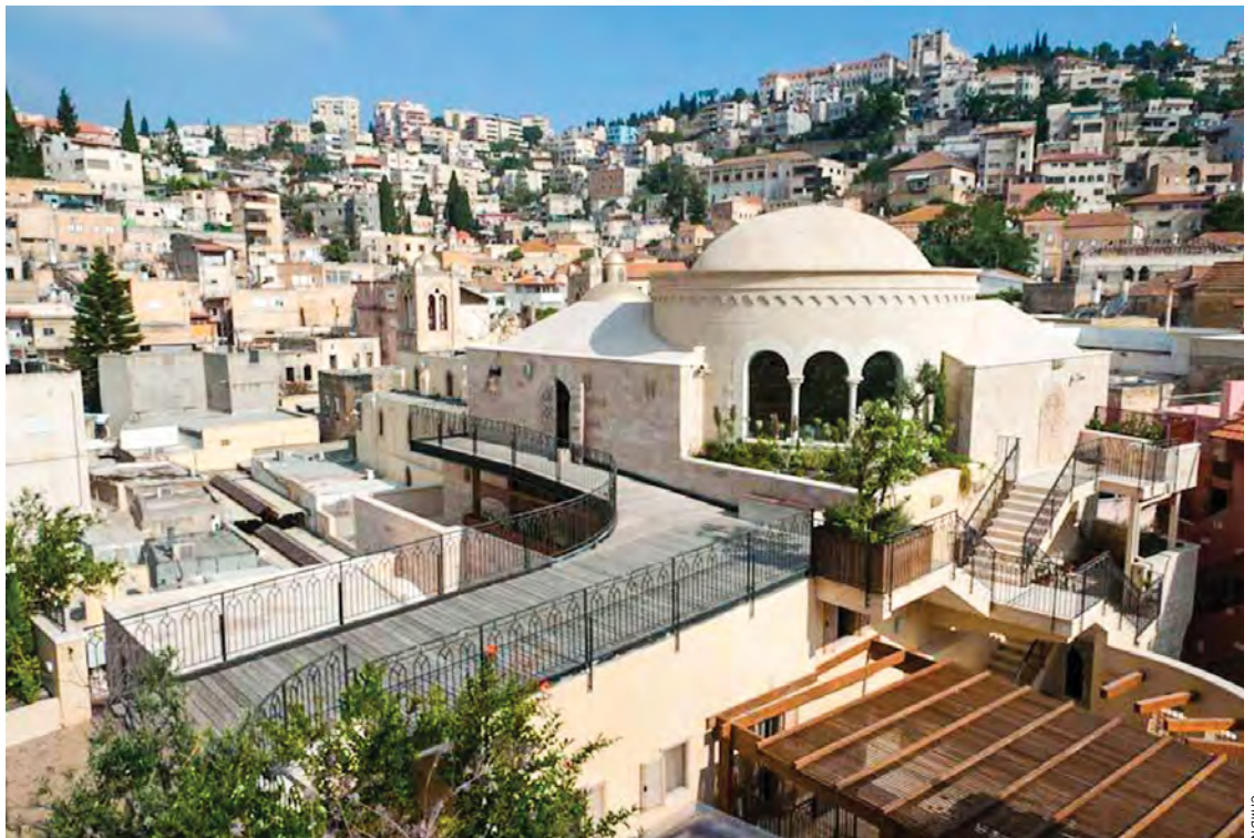
A RESCUE EXCAVATION done in 2009 prior to the construction of the International Marian Center, pictured here, revealed the remains of another first-century courtyard house from the time of Jesus. Featured in the photo is the dome of the center's chapel.
