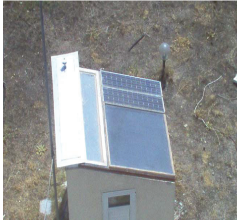
FIGURE 2. A test cell with a solar roof which consists of two c-Si PV panels while the rest of the roof operates as a solar collector.
