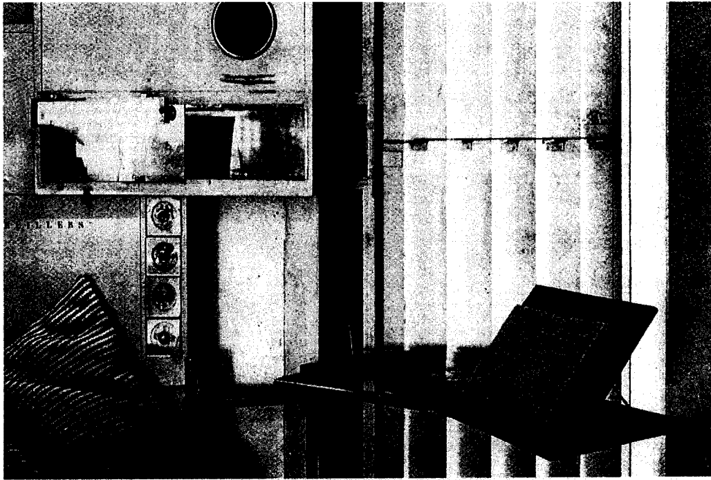
Figure 27. E.1027: alcove divan headboard with electrical outlets and built-in, pivoting bedside table.
