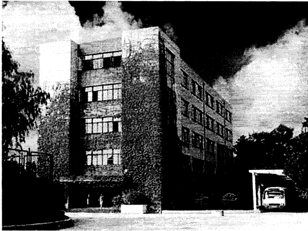
Figure 12: Education Building of VCSJTU
