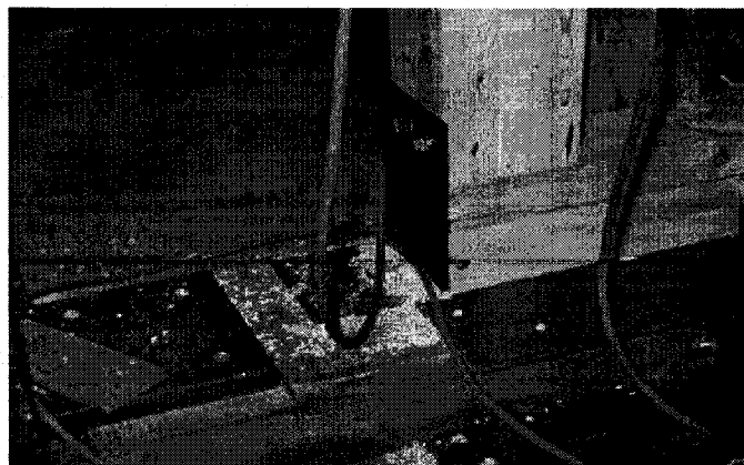
Figure 9. Additional tie-down used on Wall No. 8.
