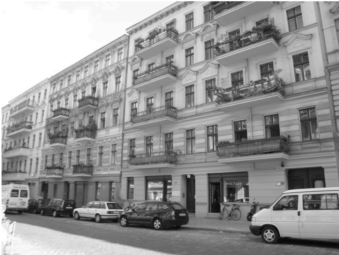
Photo 4.2: Renovated Front Buildings in a late 19 th -Century Block Development Neighbourhood (here Chamissoplatz, Kreuzberg)
