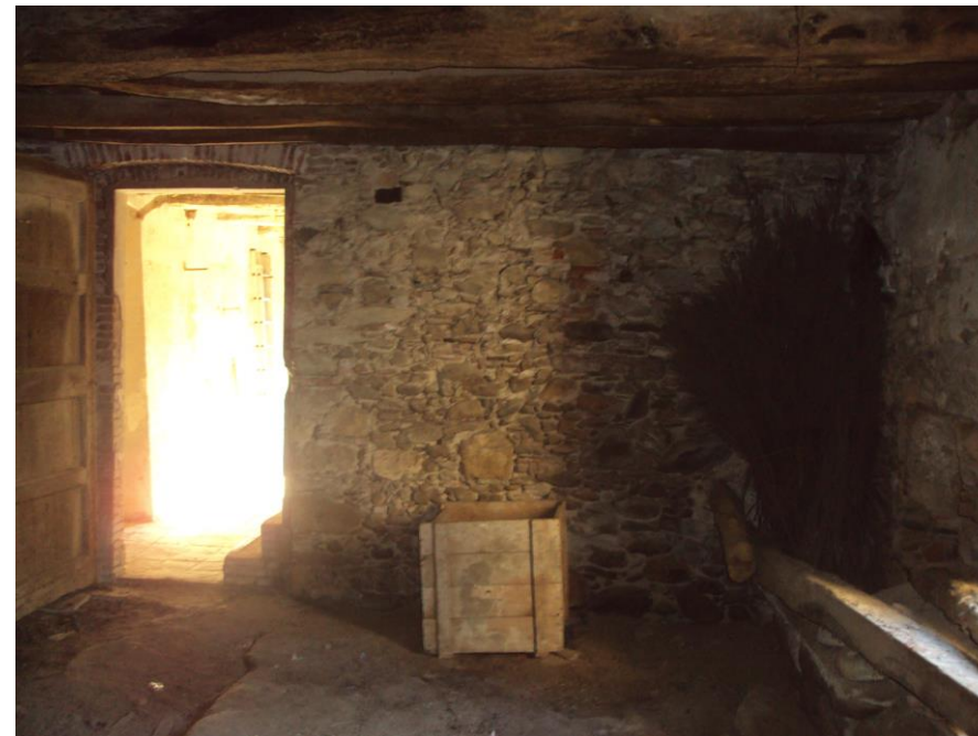
The Masonry walls seen inside
