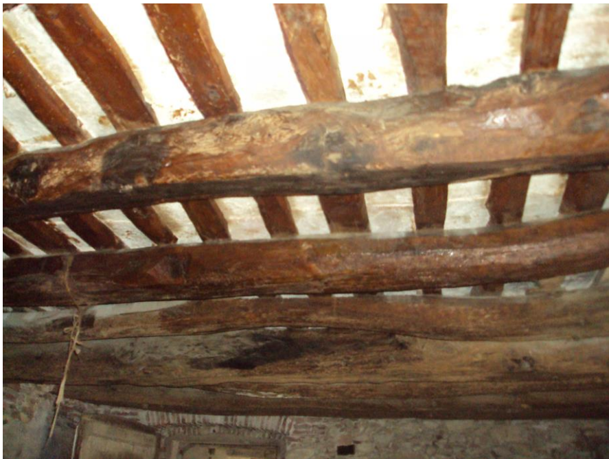
The wood Beams
