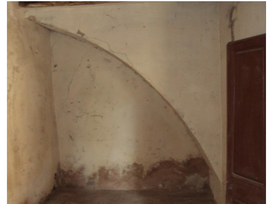
The Stairs built with brick vault plan
