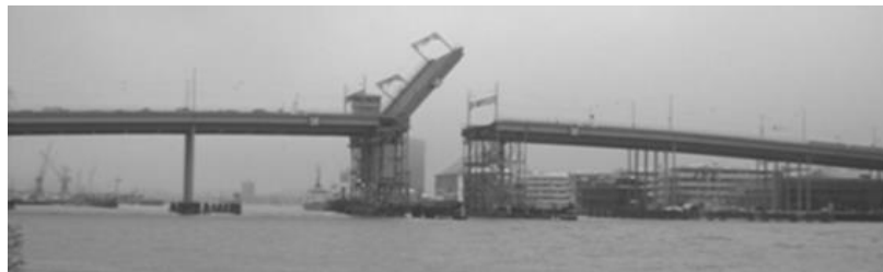
Fig. 19 The Götaälv bridge monitoring by DiTeSt system
