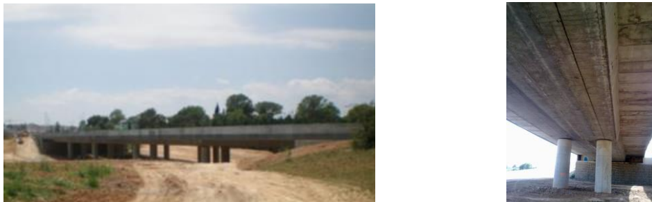
Fig. 14 Viaduct Road BP-1413 monitoring by ODiSI
