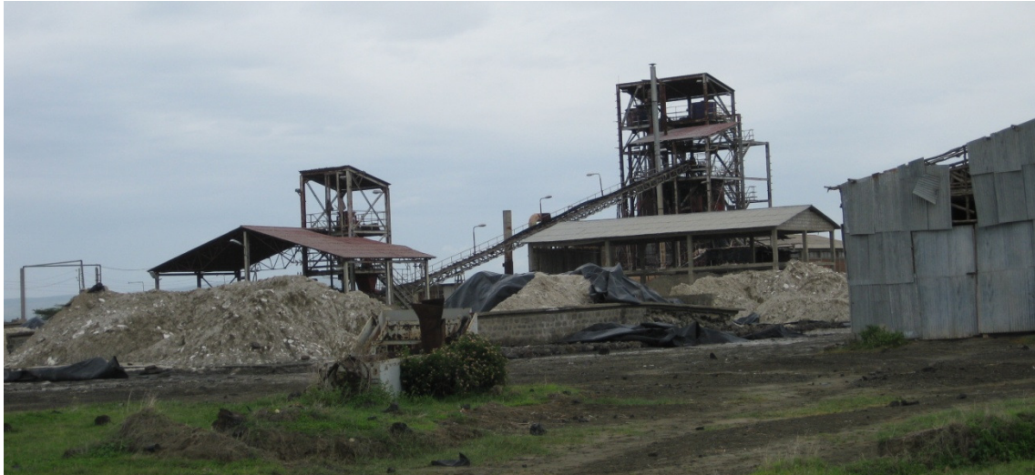
Figure 40. Soda ash factory. Author: Ester Raventós
