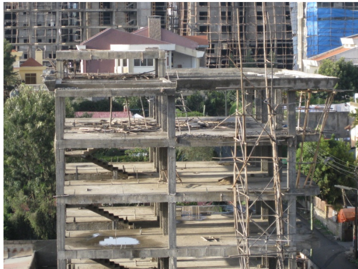
Figure 20. Scaffolding made of wood in Addis Ababa. Author: Ester Raventós
