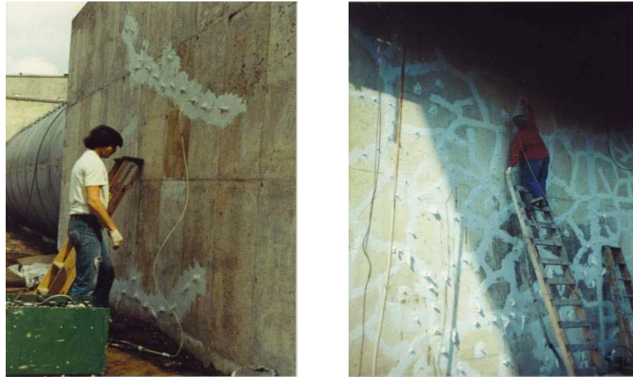
Figure 4.8 Epoxy resin injection [32]
