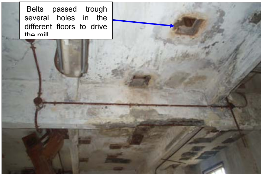
Figure 8.5 Concrete floor slab, primary and secondary beams
