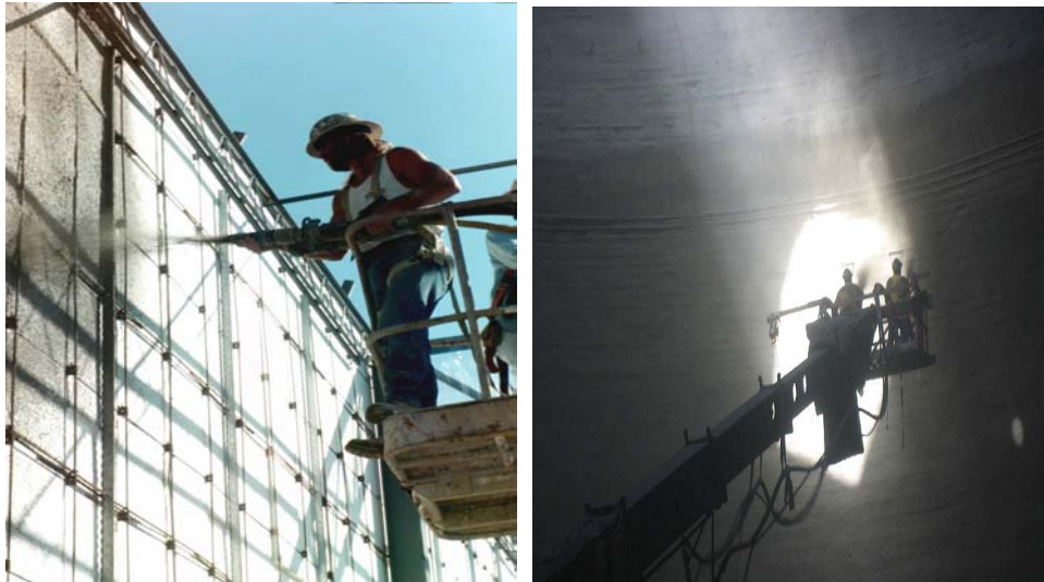
Figure 4.11 Application of shotcrete on external wall and inside of dome
