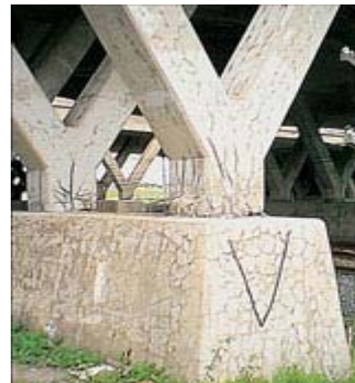
Figure 2.34 ASR-Induced Damage in Restrained Concrete Elements [26] and [27]
