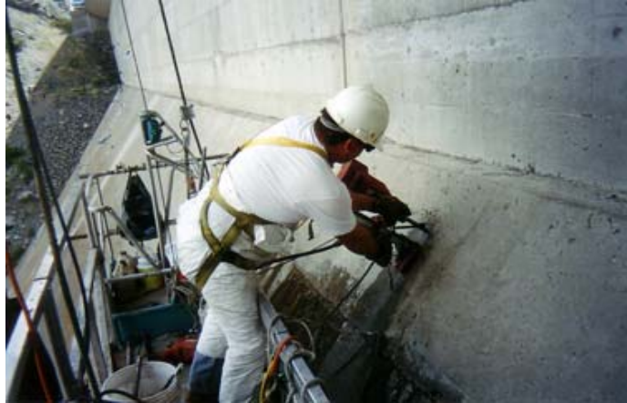
Figure 4.7 Application of chemical grout [31]
