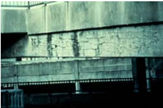
Figure 2.34 ASR-Induced Damage in Restrained Concrete Elements [26] and [27]
