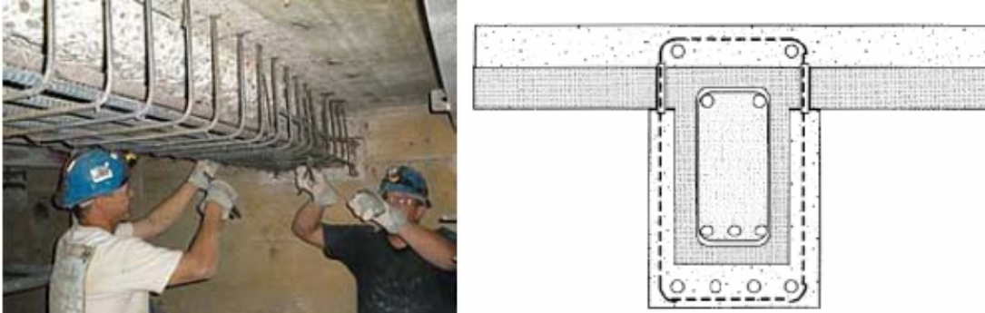
Figure 4.19 addition of steel reinforcement and concrete overlay [17]
