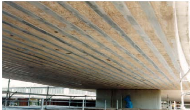
Figure 4.16 externally bonded plates using FRP [21]
