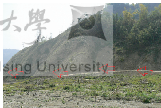
(f)小林村對岸內凹邊坡突出山脊處
