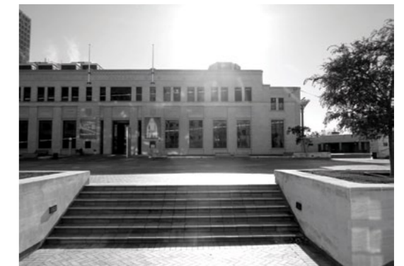
1.4 City Gallery, 1940. (2011). Civic Square, Wellington. Source: Authors own photograph
