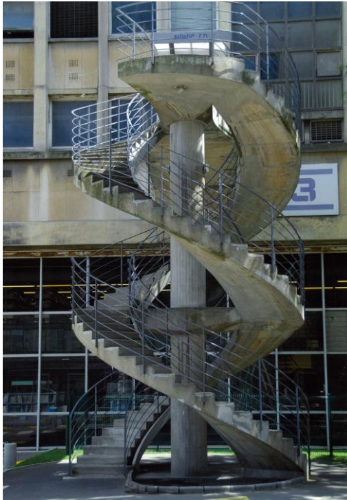
Figure 3.19: Double-Helix Staircase, Place Jussieu 4, Paris
