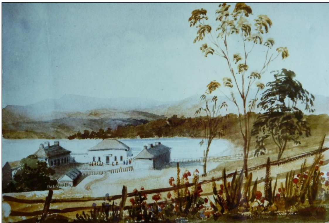
Figure 3-6: Illustration from ca.1841 looking south over the completed prisoners' barracks (Owen Stanley, Penal Settlement VDL, Convict prison near the Coal Mines , n.d. [January 1841], Tasmanian Museum and Art Gallery)
