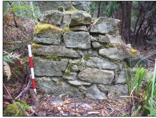
Feature 12, showing north-facing elevation, looking S
