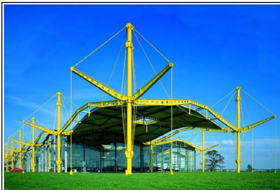
Figure 23. Renault Distribution Centre. (Photograph: Foster and Partners, http://www.fosterandpartners.com )
