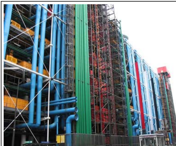
Figure 20. Centre Pompidou, Paris. (Photograph: http://www.rsh-p.com/ )
