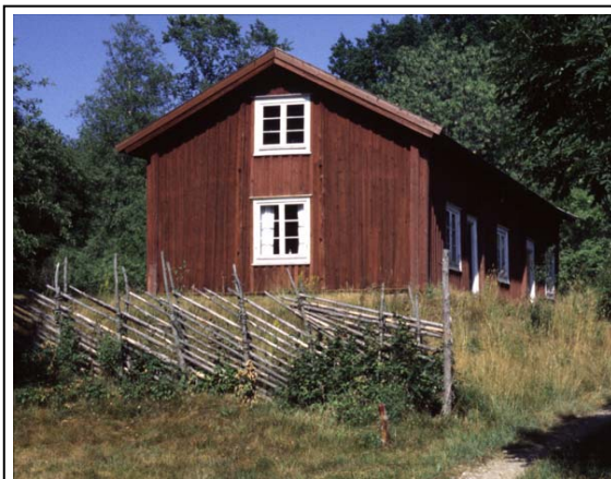
Figure 24. A red timber cottage in rural Sweden. (Photograph: C. Hagerhall)
