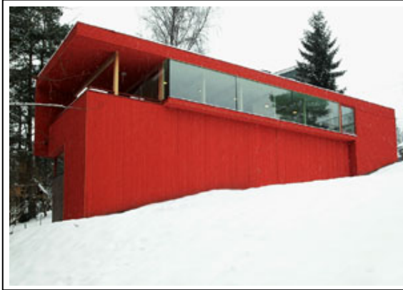
Figure 22. The Red House, Norway. (Photograph: Nils Peter Dale, http://www.jva.no/ )
