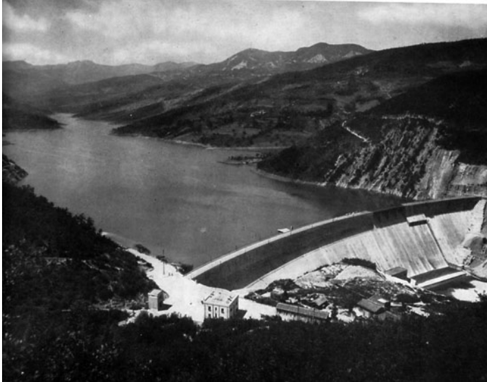
Figure 5.5. Picture of the Mignano dam taken in 1953 (in [2]).
