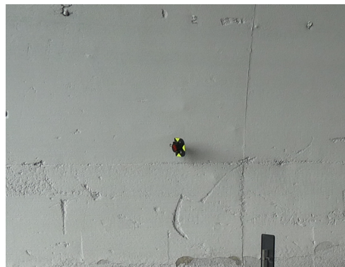
Figure 4: Example of additional benchmark materialized on the tunnel wall
