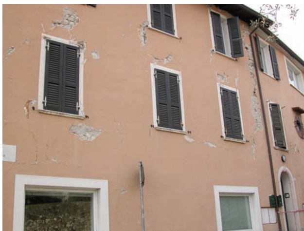
Foto 3-4 Lesioni diffuse a edifici in muratura a Salò e Pavone. Photos 3-4 Extensive cracks on masonry buildings in Salò and Pavone.
