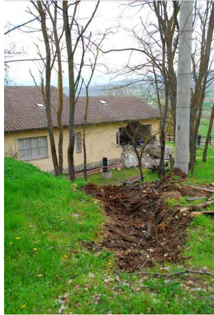
Figure 115. Last impact mark prior to impacting building at the Caves of Stiffe; the block trajectory was above the small tree (42.255N 13.547E).
