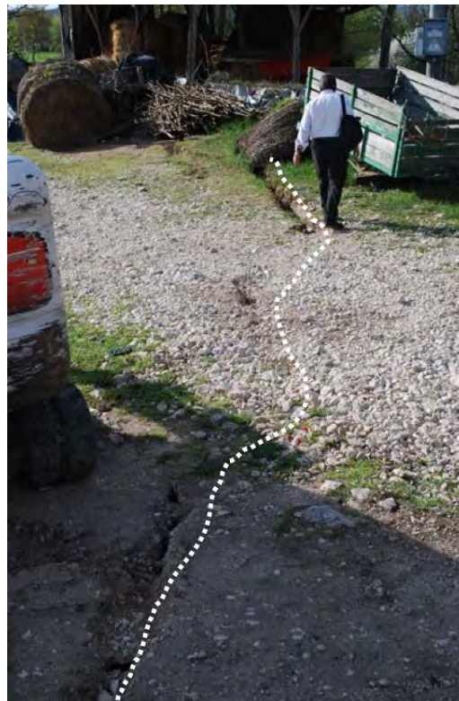
Figure 143. Ground cracks up to 1.0 m deep, 20 m long, and with maximum of 15 cm vertical displacement (down-dropped toward river) developed directly adjacent to bridge abutment (42.324N, 13.478E).
