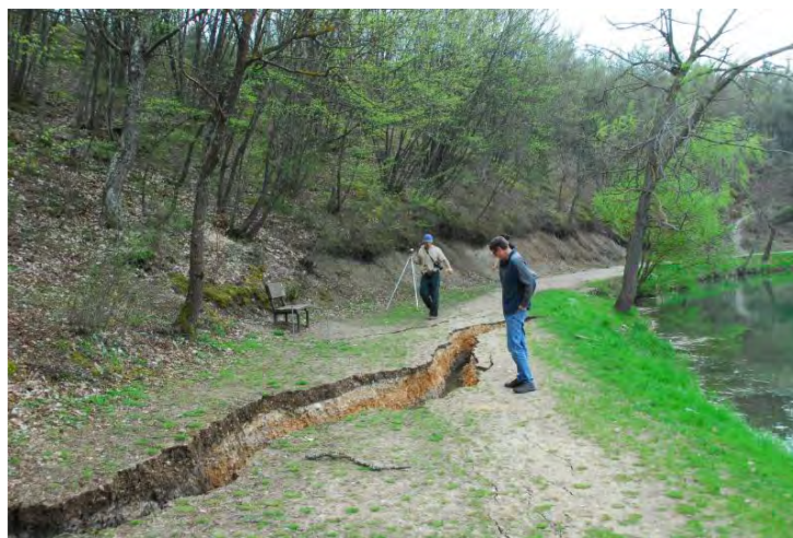
Figure 159. Ground cracks along the eastern perimeter of Lake Sinizzo (42.291N, E13.576).
