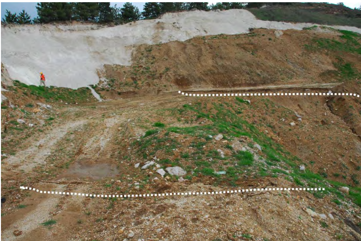
Figure 150. Graben structure (between lines) created by parallel down-dropped shears (42.435N, 13.330E).
