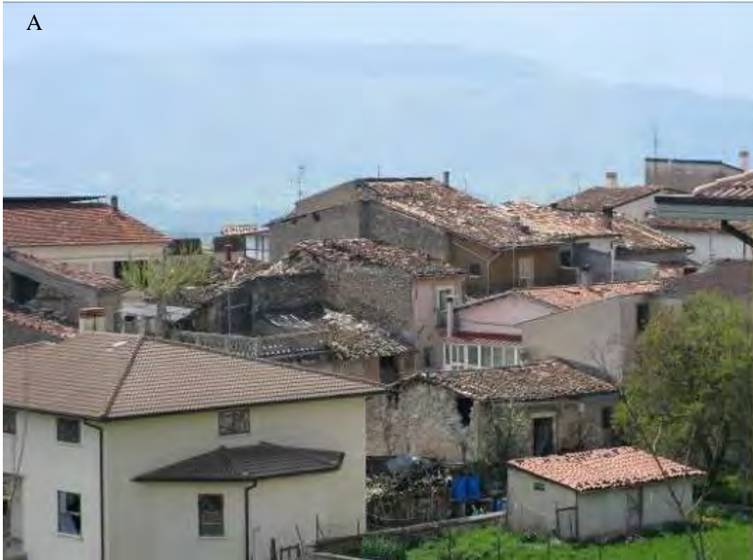
Figure 86. Poggio Picenze. (A) Variable damage (D3-D4) on masonry buildings of different style.
