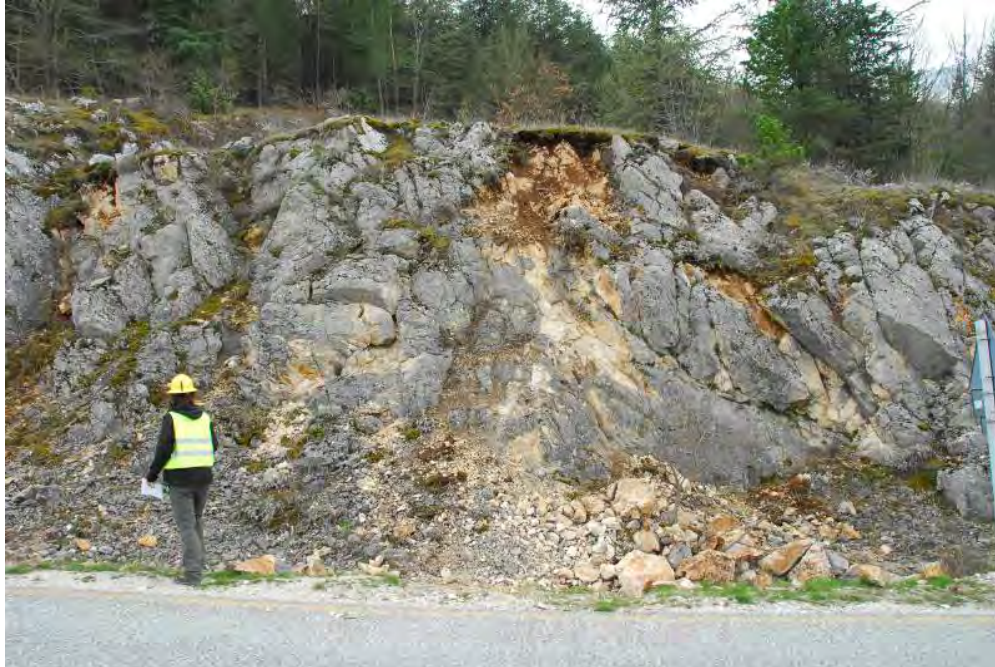
Figure 117. Shallow ravelling-type failure of weathered limestone blocks (42.278N, 13.467E).
