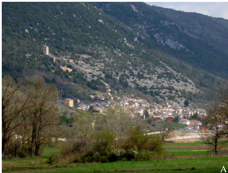
Figure 61. (A) The village of San Pio delle Camere built on Mesozoic limestone. This picture was taken from the lower flanks of Castelnuovo (from location 42.2898°, 13.6297° looking southeast).
