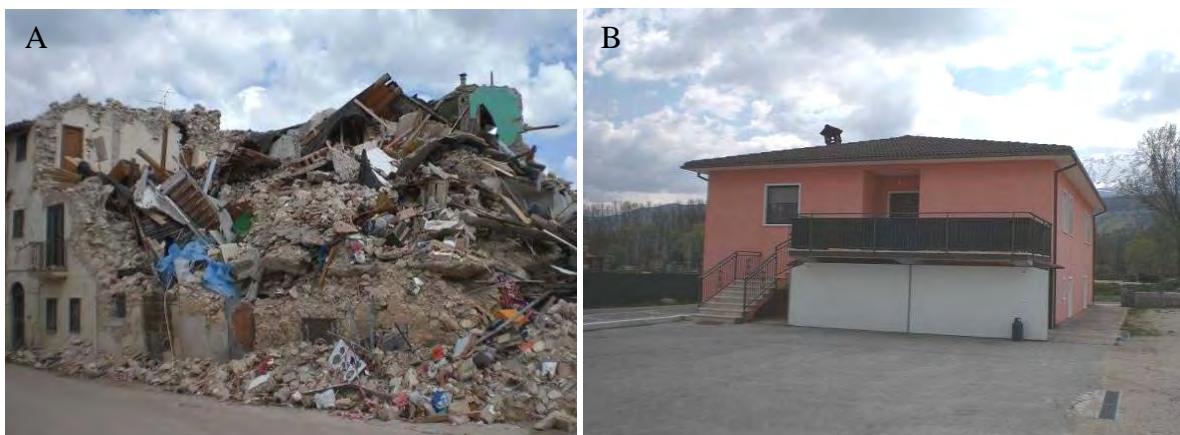
Figure 67. Onna. (A) D5 damage level on masonry building structures, (B) D0 damage on a RC building (except for the tilting of the chimney).
