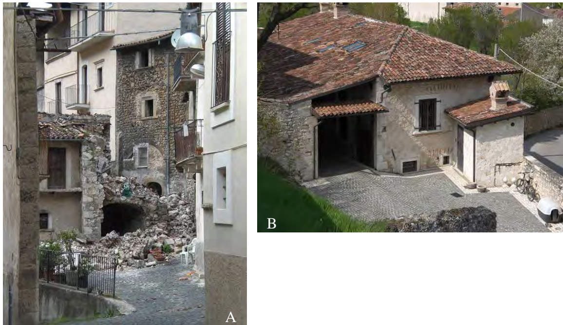
Figure 77. Fossa. (A) Collapse of masonry constructions in the historic center, (B) Strengthened masonry construction with no damage.
