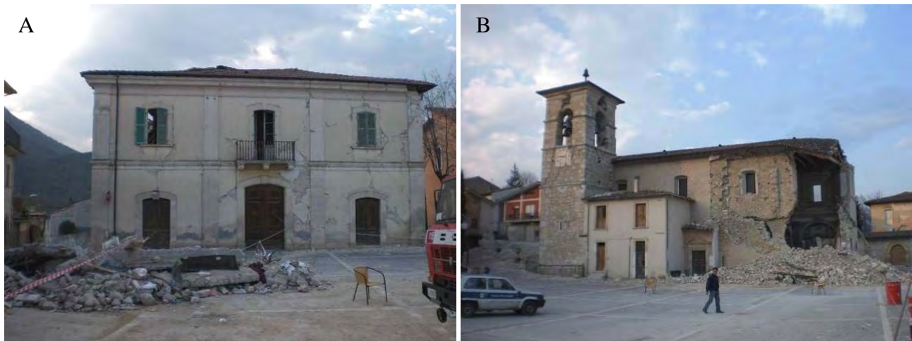
Figure 89. Villa S. Angelo, historic center with (A) masonry building crack,; (B) partly collapsed church.
