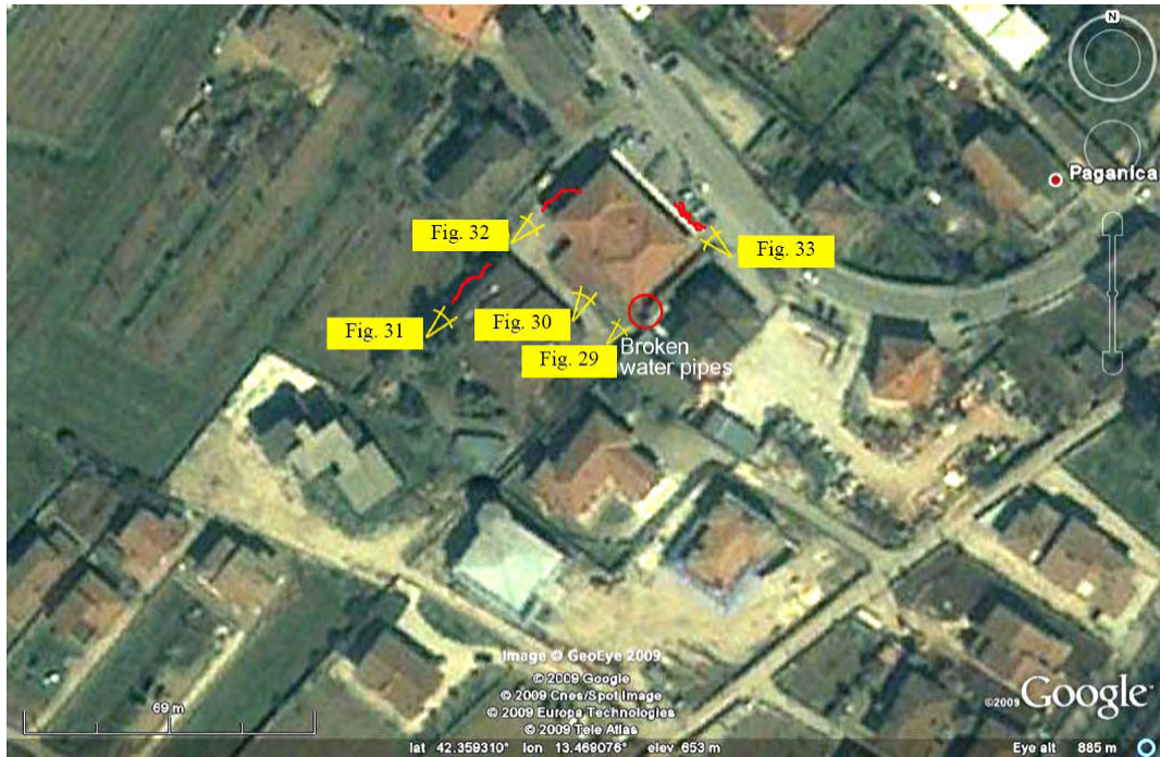
Figure 28. Plan view of Paganica site with marked positions of ground fissures, paved walkway cracks and broken water pipes. Directions of photo shots are indicated by yellow signs.
