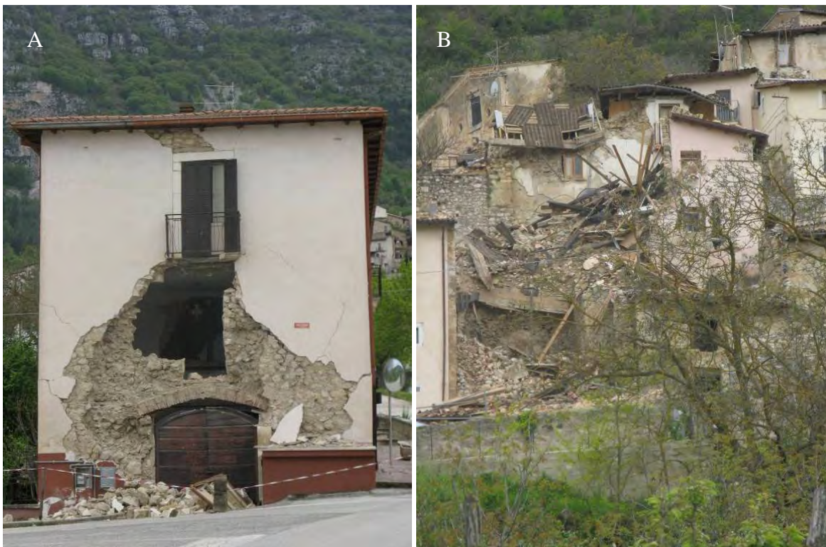
Figure 82. Casentino. (A) Partial collapse of the masonry building at the entrance of the village, (B) Collapse of old poor quality masonry buildings in the historic center.
