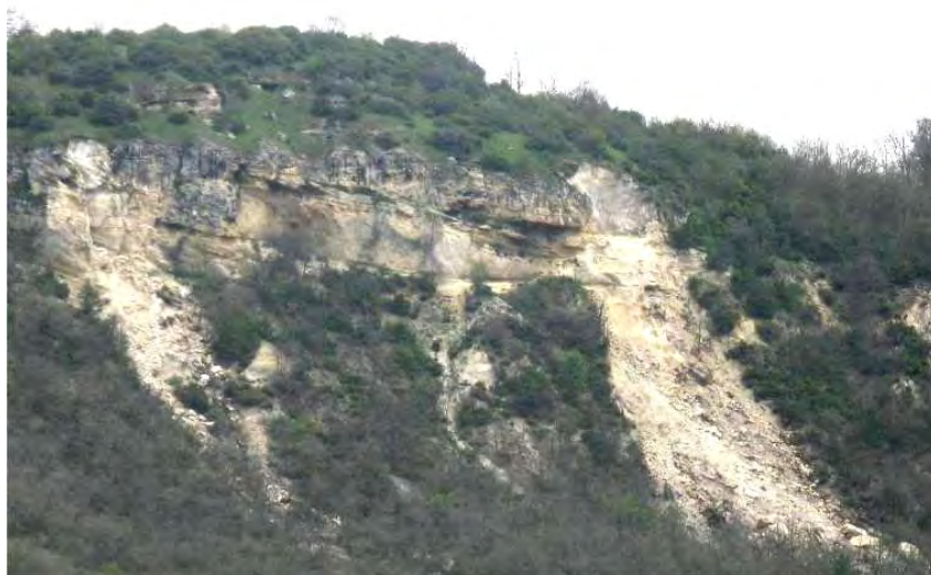
Figure 120. View of the cliff overlooking the northeastern side of Lake Sinizzo. Two failures in the overhanging thick layers of conglomerates are apparent with the related rock avalanches (42.292N, 13.580E).
