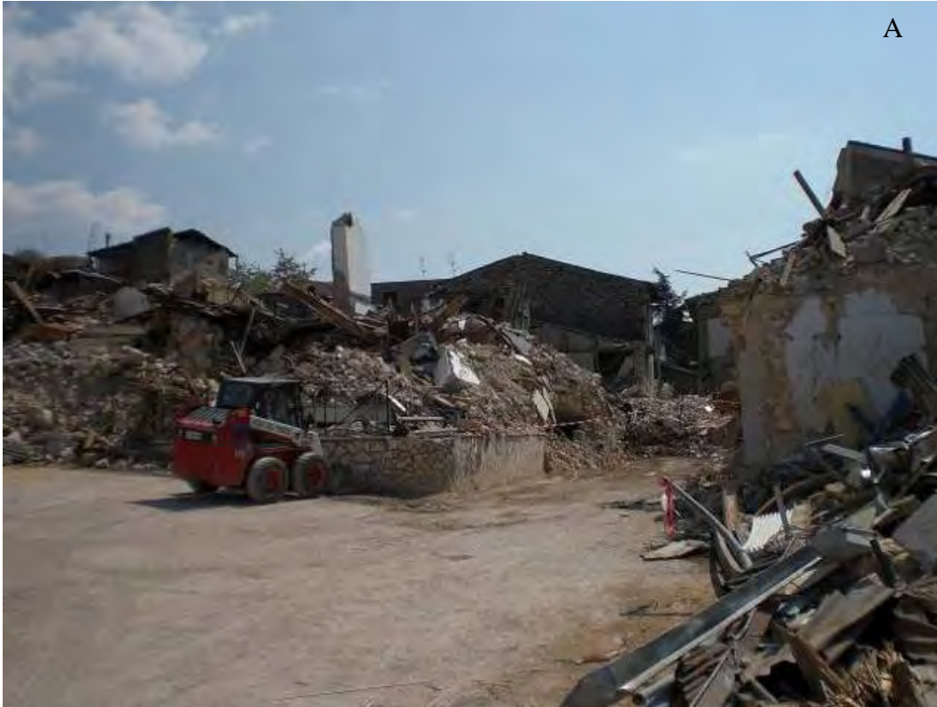
Figure 72. San Gregorio. (A) View of the historic center with collapsed masonry buildings.
