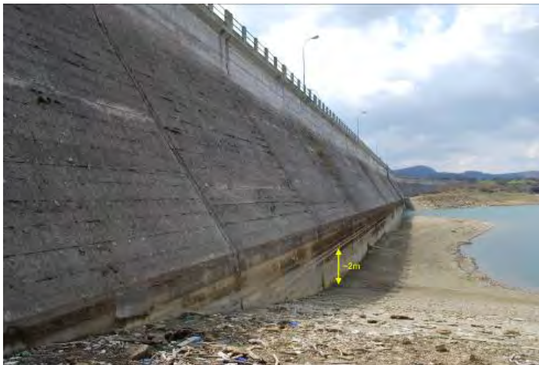
Figure 178. Upstream face of Sella Pedicate dam. The lowering of water level decided by ENEL following the main shock is evident in the photo (42.514954°N, 13.369194°E).
