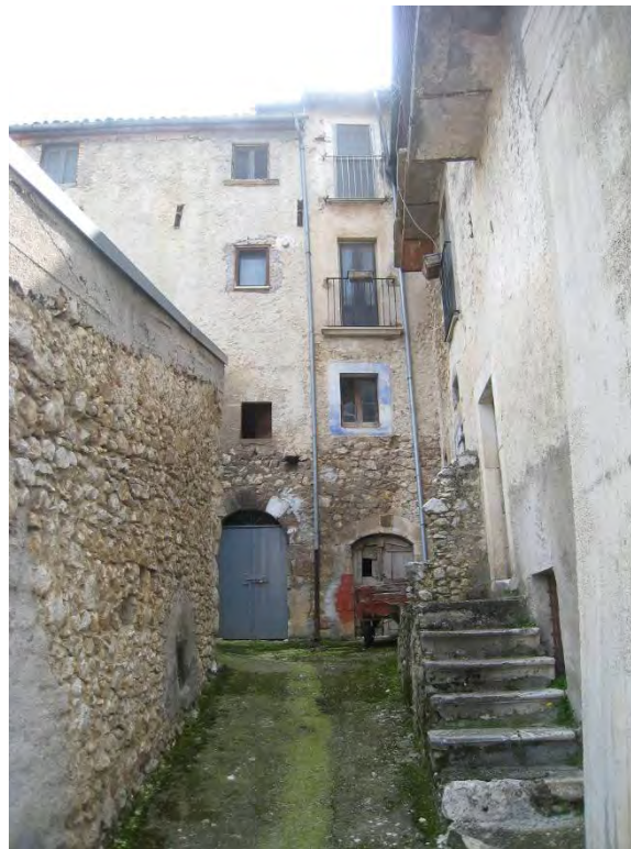
Figure 63. The reconnaissance team observed no damage to the town of Tussio. The town is built on Mesozoic calcareous bedrock (42.2657°, 13.6414°).
