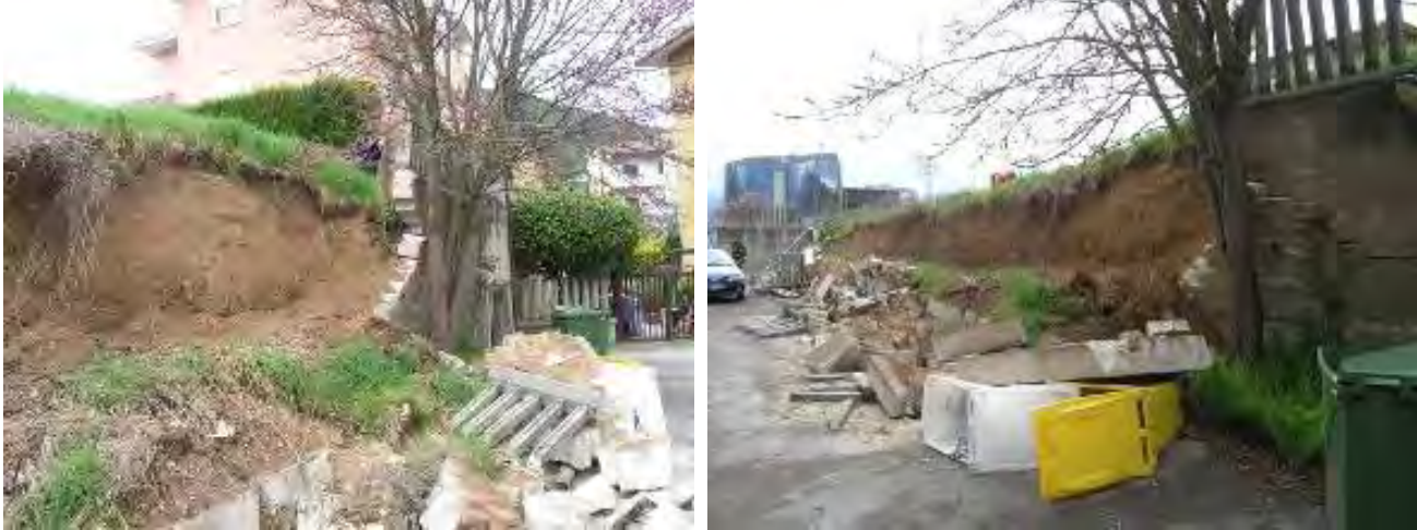
Figure 193. Toppling of masonry retaining wall at the outskirts of L'Aquila (42.366803°N, 13.376561°E).
