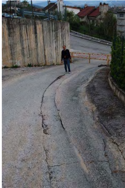
Figure 155. Seismic compression of trench backfill in the town of Paganica (42.365N, 13.465E).
