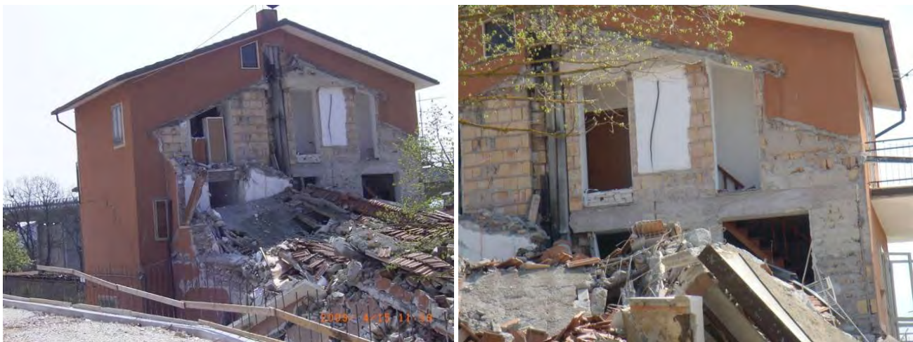
Figure 104. Masonry structure at waypoint GB-82-1.
