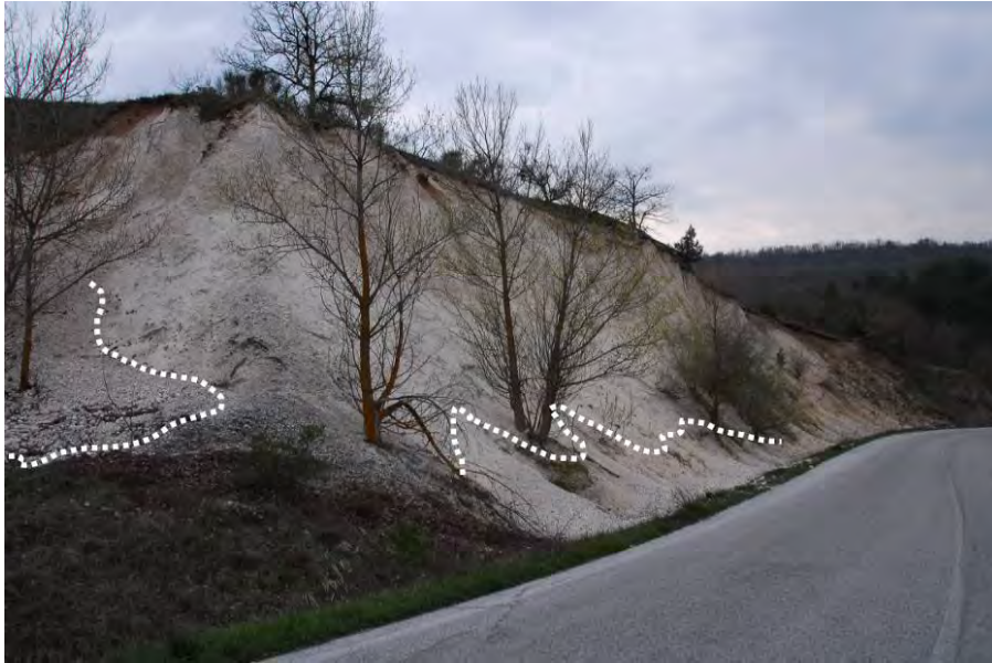
Figure 121. Minor ravelling of weakly cemented sand and gravel; dashed lines indicate the extent of freshly deposited talus along the base of road cut (Via Opi N42.261, E13.581).
