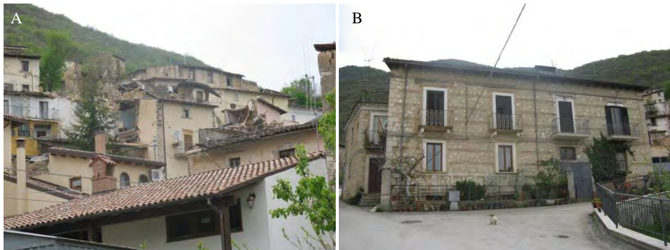
Figure 90. Tussillo. (A) View of the historic center with some collapsed masonry buildings on the background, (B) Masonry building at the entrance of the village showing no damage.
