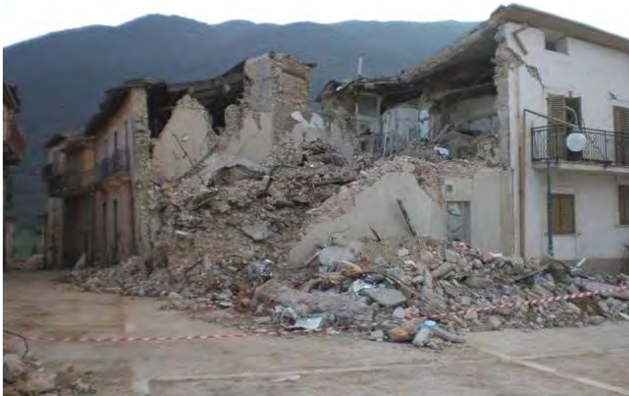
Figure 88. Villa S. Angel. (A) Collapsed masonry buildings (D5) in the historic center.
