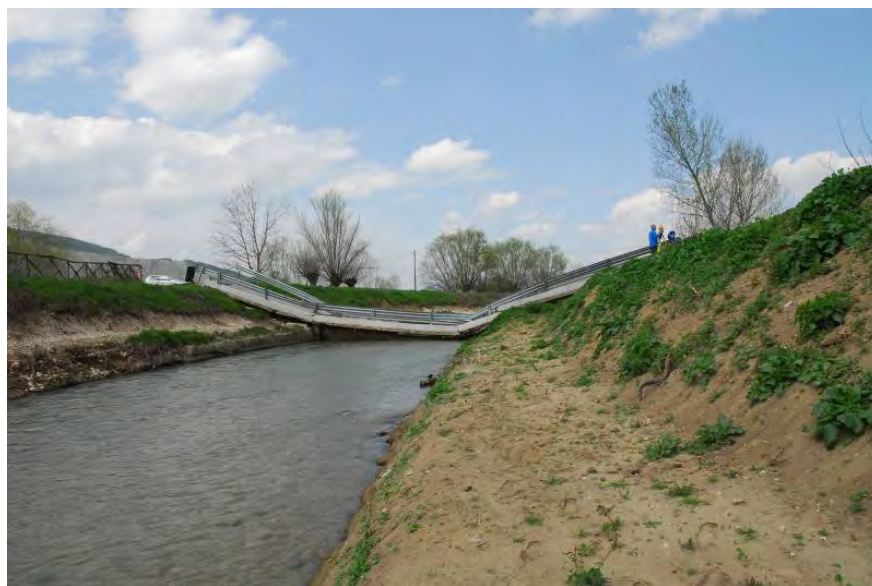
Figure 147. Flood protection levee in vicinity of bridge collapse (42.325N, 13.463E).
