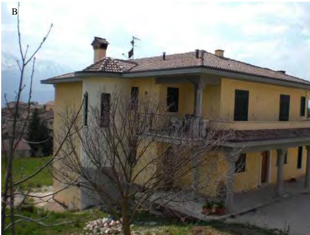
Figure 86. Poggio Picenze. (B) Undamaged RC house (D0) close to the (C) monumental church (D3).
