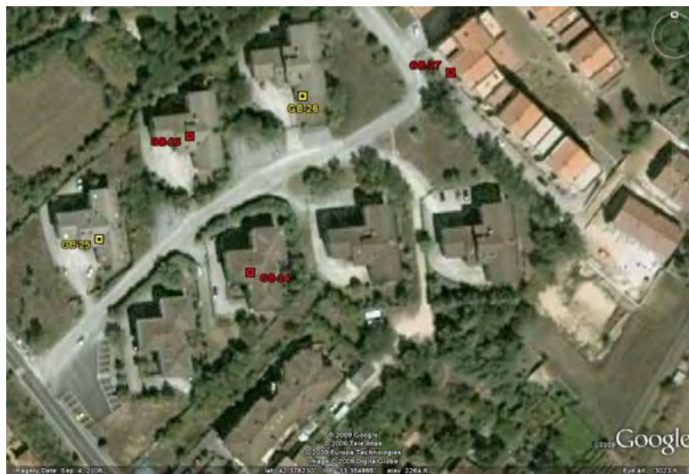
Figure 108. Cluster of damage in zone (d).
