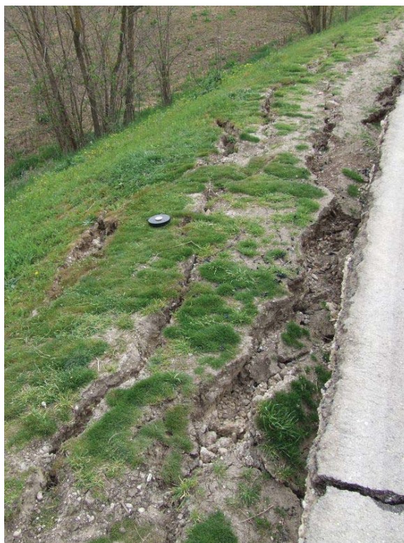
Figura 53 Dissesti ai margini del manto stradale, WPT RN8, 42.3233/13.4777. Figure 53 Sliding and spreading on the roadside, WPT RN8, 42.3233/13.4777.
