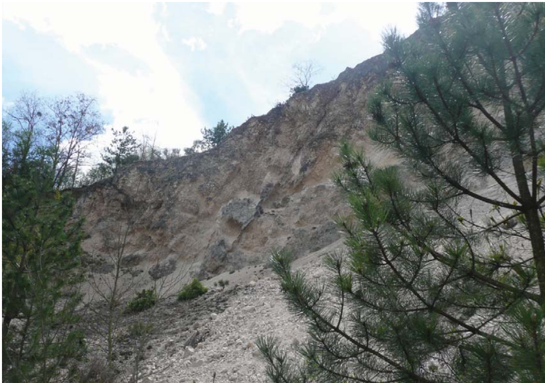
Figura 43 Faglia nella cava di Fossa (WPT LC63, 42.3003/13.4847). Figure 43 Fault in the quarry near Fossa (WPT LC63, 42.3003/13.4847).
