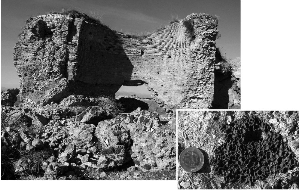
Fig. 1. Baths at Anazarbos with scoria in vaults. 150x95mm (300 x 300 DPI)
