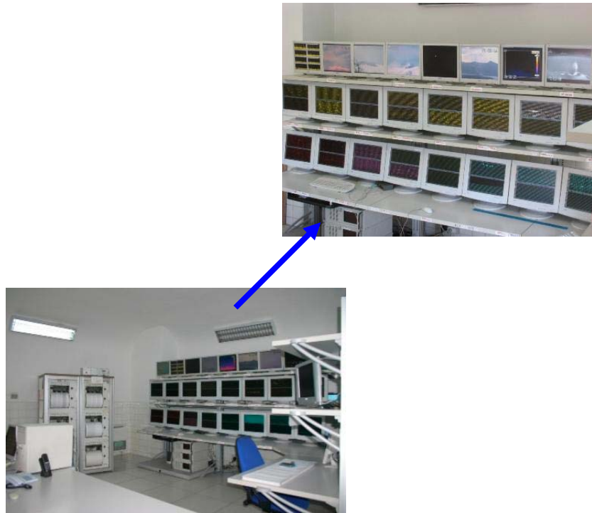
Fig 1. The Control Room inside INGV in Catania
