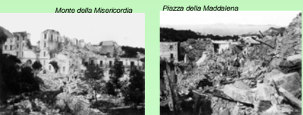
Damage at Casamicciola, upper part by Achille Mauri
