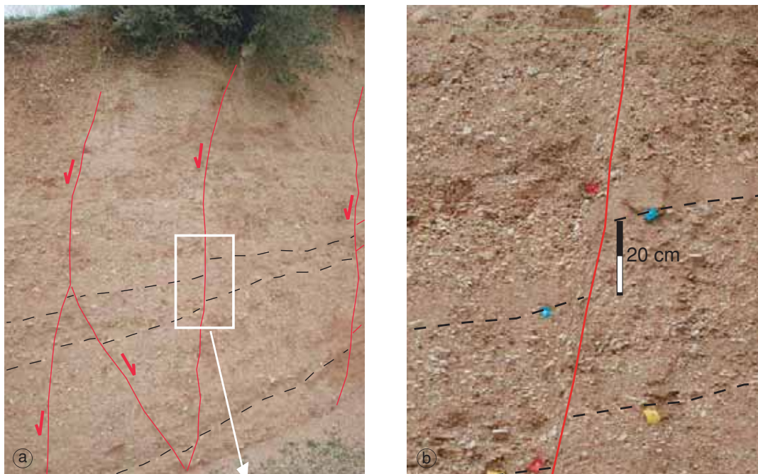
Fig. 14a,b. a) Photo of the NW wall of the artificial cut affecting the slope debris near the Gubbio Fault. In figure are highlighted normal faults (continuous line) and main depositional horizon (dot line); b) detail showing the re-oriented clasts and the offset amount.
