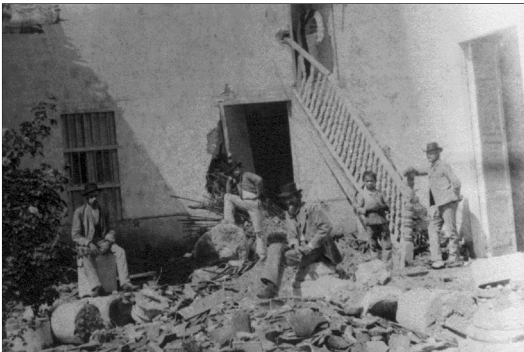
Fig. 3. Damage caused by the earthquake of 1894 in Mérida, Venezuela (from Romero, 1894).
