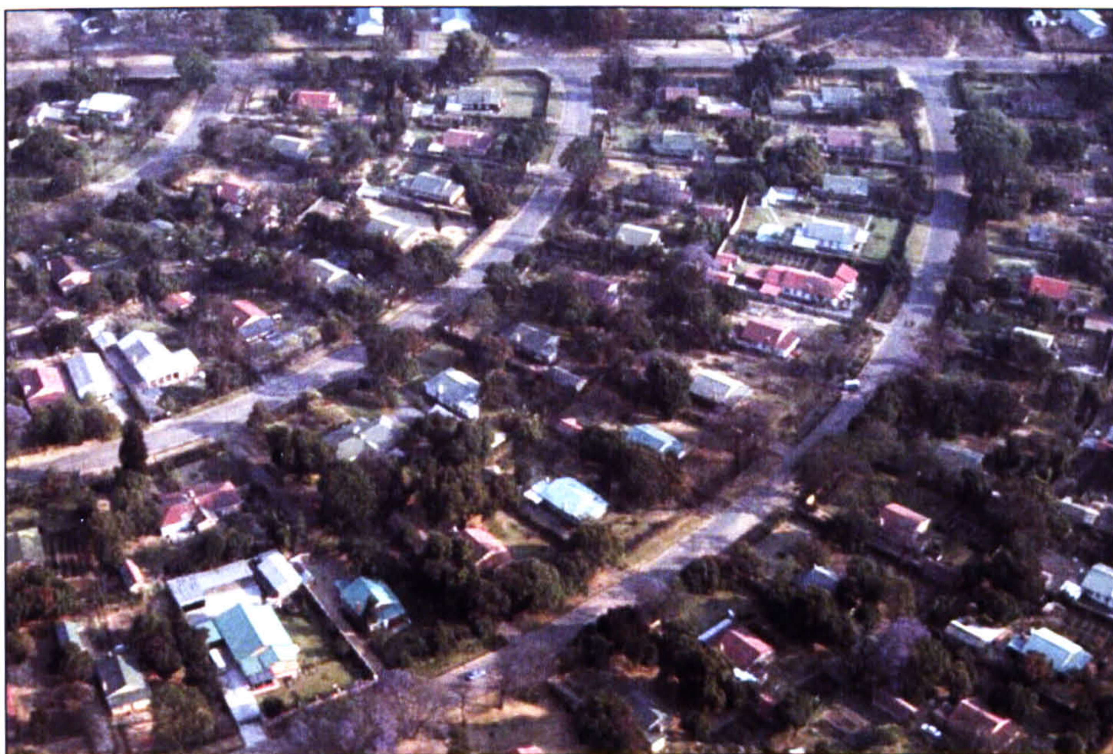
Figure 5.2: An aerial photograph taken in July 2005 of a former European township (now referred to as a ‘high cost township’) in the town of Chingola built circa 1950
