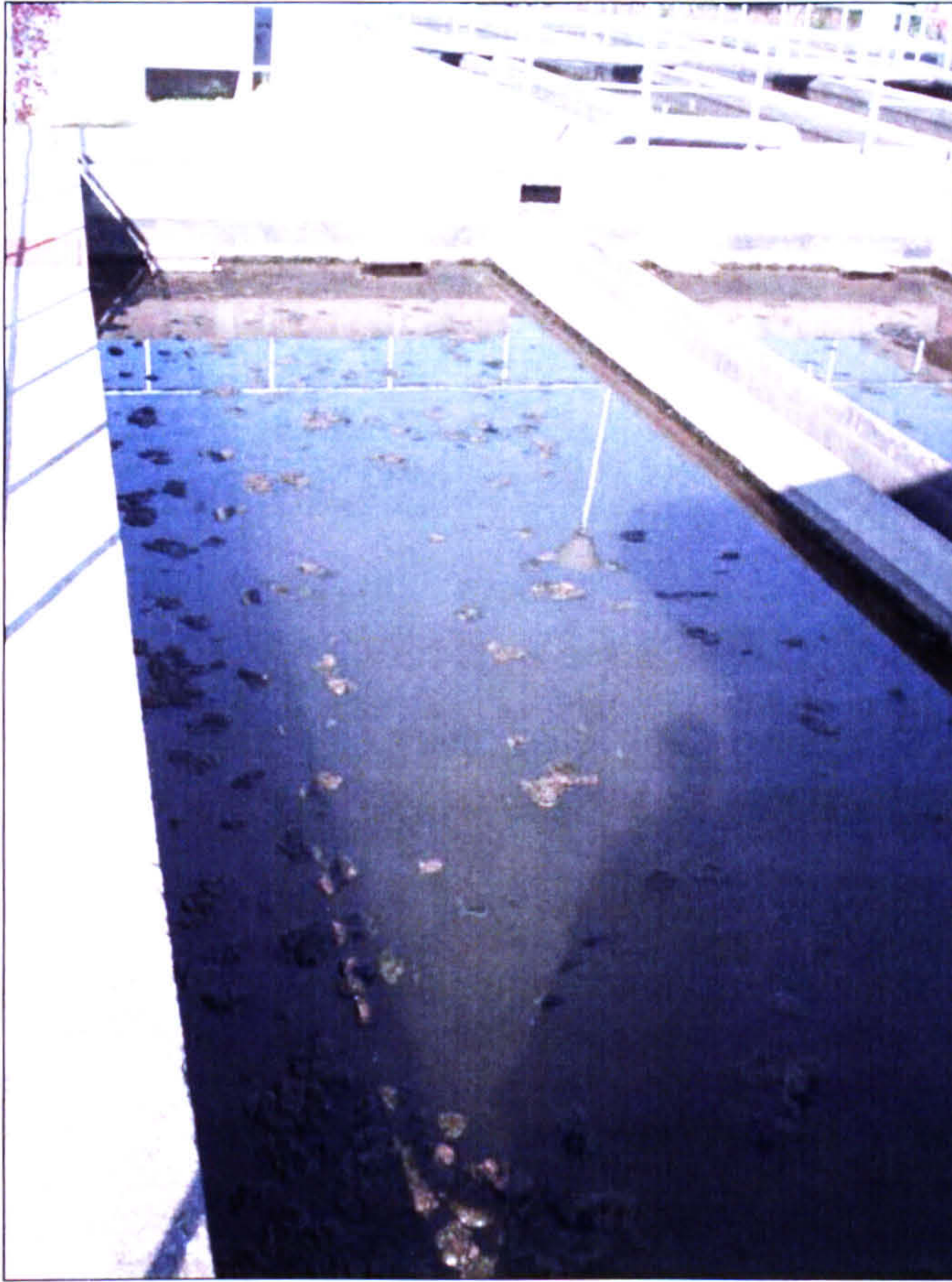
Figure 7.13: The accumulation of algae at the Chingola water treatment plant in May 2005
