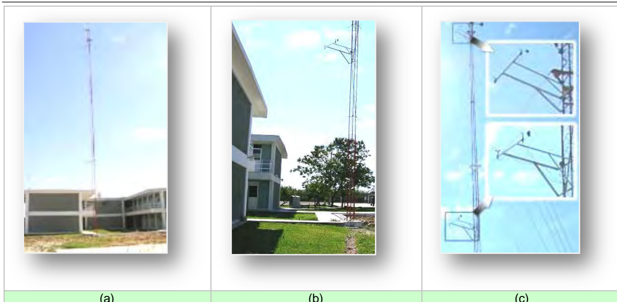
Figure IV.2. Images of the measurement tower: (a) overall view from the westerly direction, (b) view from the northerly direction showing the tower base, (c) close up view from the northerly direction showing the position of the installed sensors.
