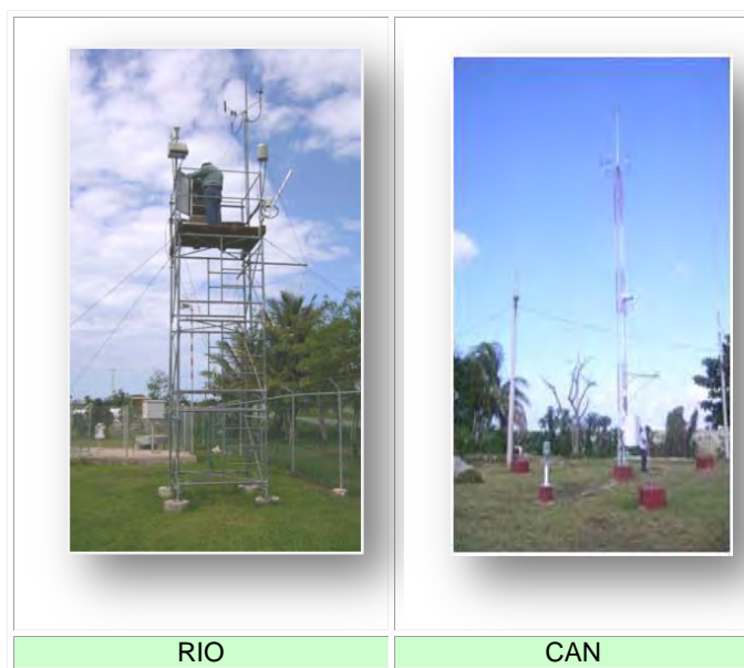
Figure III.3. Photos showing the two types of meteorological measuring structures used at the study sites (Type A: Scaffolding and Type B: Tower), in these cases, the RIO and CAN stations.
