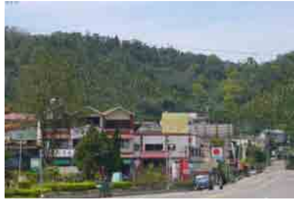
the provincial highways No. 21 in Yuchi
