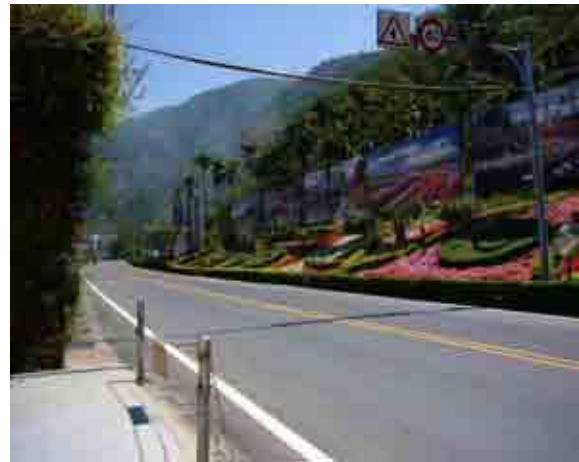
the provincial highways No. 14 in Puli
