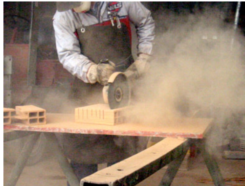
Fig. 74: Dry cutting of brick with a wheel cutter
