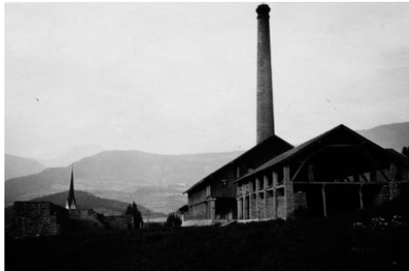
Fig. 36: The Vereinigte Pustertaler Ziegelwerke brick plant around 1925. In the foreground the naturally vented dryer and in the back the building hosting the Hoffmann kiln
