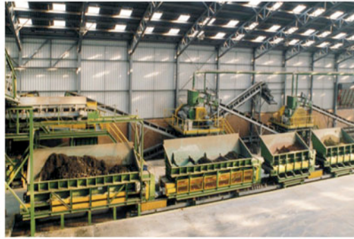
Fig. 6: Handle box feeders in a modern brick plant around 1985
