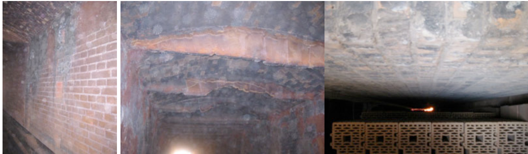
Fig. 42: Ziegel Gasser Mattoni GmbH S.r.l. vaulted roof tunnel kiln
