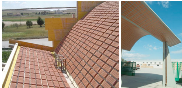
Fig. 26: Shaped brick structures
