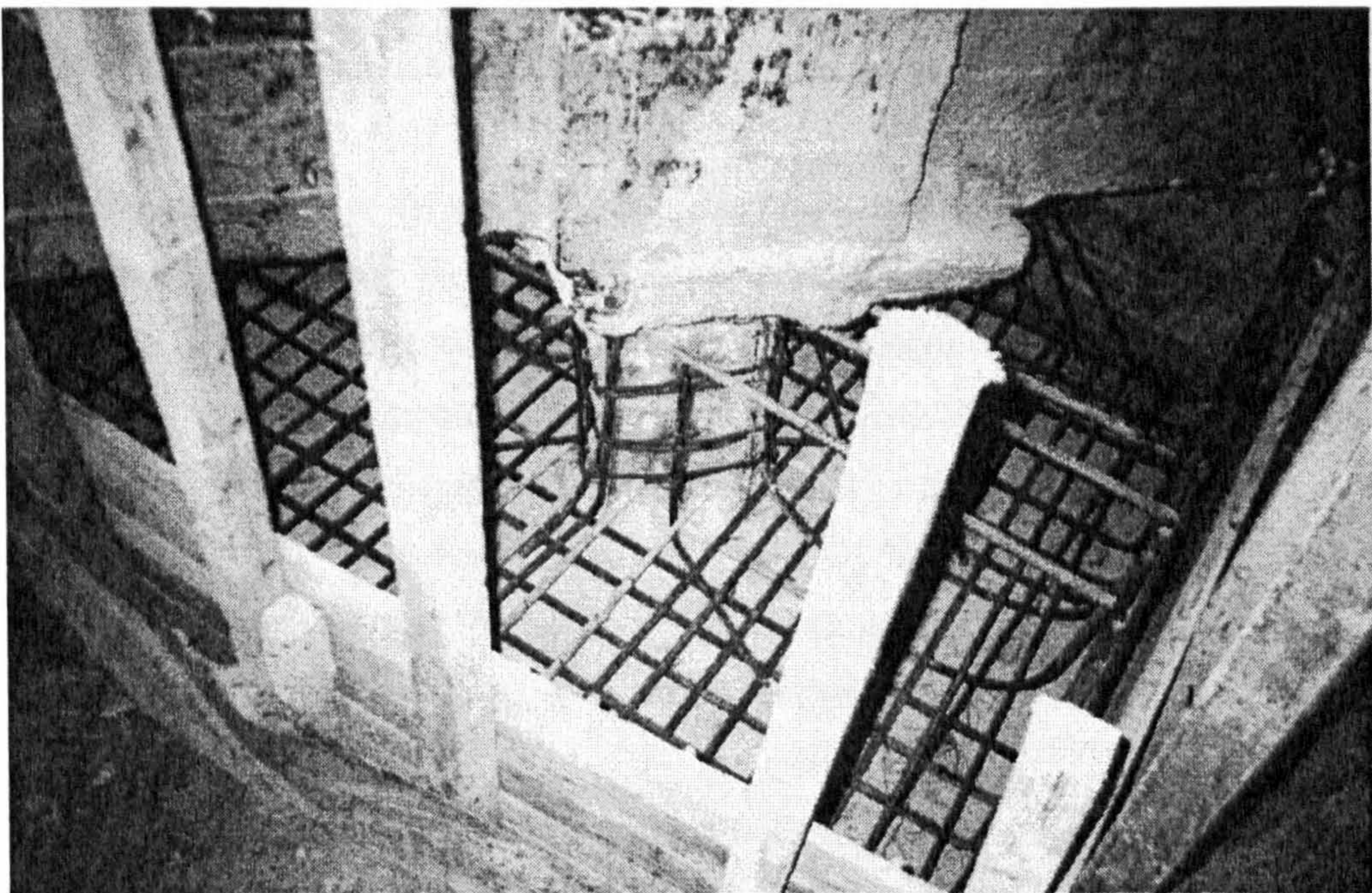
Figure (7.9) Amending foundations problems
