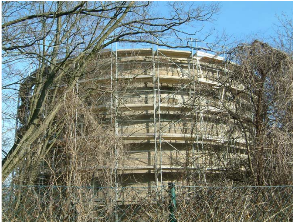
Part of Speer's Great Arch, 1941. This 'ignored' remnant sits on the corner of Loewenhardtdamm & General-Pape-Strasse (Photograph taken by author, 02.07)
