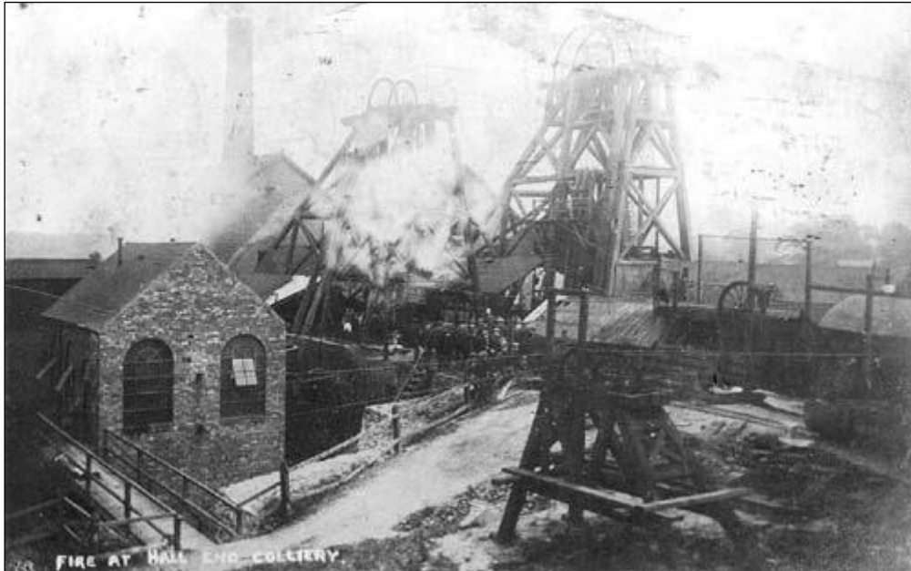
Illustration 3:2 A Fire at Hall End Colliery 1910. 142
