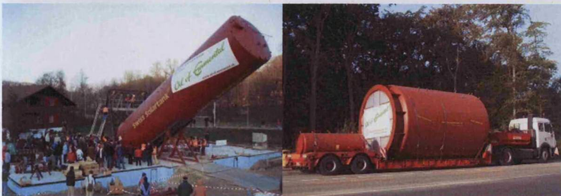
FIGURE 12: IMAGES FROM JENNI. FITTING THE STORAGE PRIOR TO BUILDING CONSTRUCTION (LEFT). TRANSPORTATION OF A 60CB.M WATER TANK (RIGHT) (WWW.JENNI.CH).
