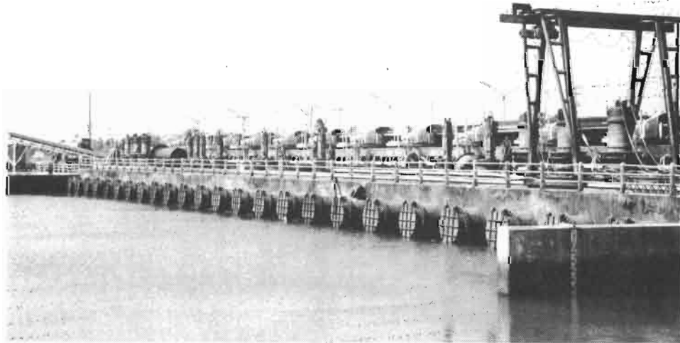
PHOTO. 2 SLUICE GATE AT CHAROEN RAT, DECEMBER 24, 1999.
