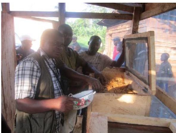
Photo 23: Joint installation of experimental dispositive
