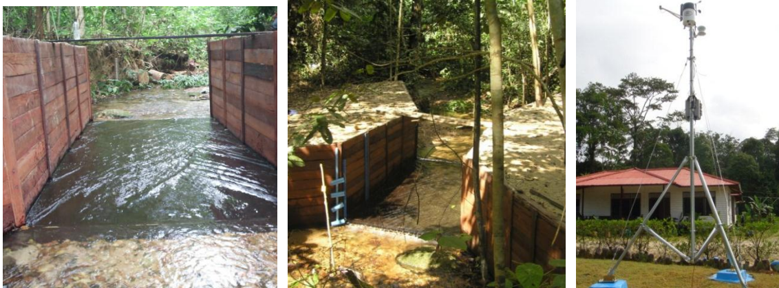
Figure 2.16 Flume weir in the C1 outlet and the weather station.
