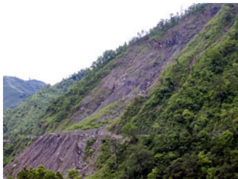
Figure 1.6 Krishnabhir in 2006, after the bio-engineered slope stabilization ( Photo Courtesy: http://www.nepalitimes.com )
