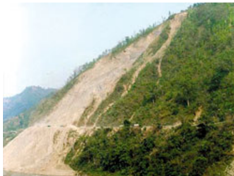
Figure 1.5 Slope failure in Krishnabhir in 2000 ( Photo Courtesy: http://www.nepalitimes.com )
