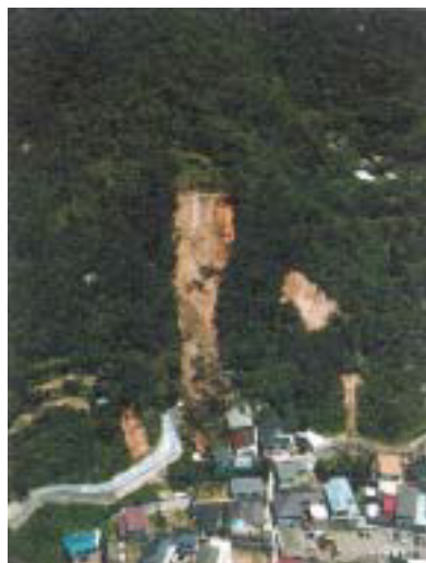
Figure 1.9 Slope failure in Uenoyama Area in Kozushima Village (July 2000, Kozushima Village, Tokyo) ( Photo Courtesy: MLIT, Japan )
