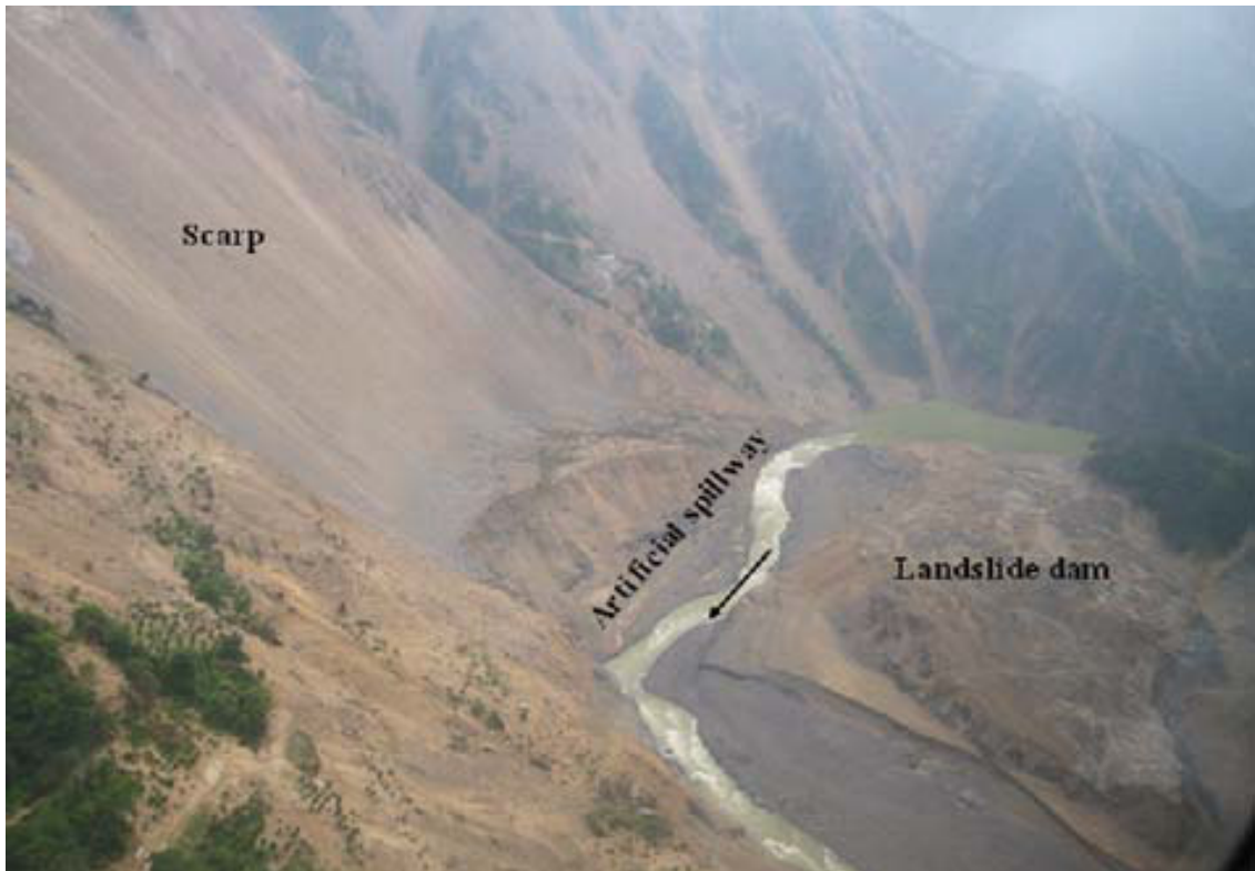
Figure 1.1 Helicopter view of the artificial spillway in the Tangjiashan landslide dam (Source: Xu et al., 2009)
