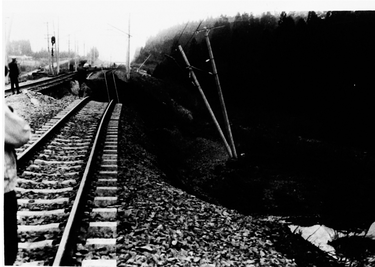
Fig.7 Rotating slide in the Tokachioki earthquake, May 16, 1968.
