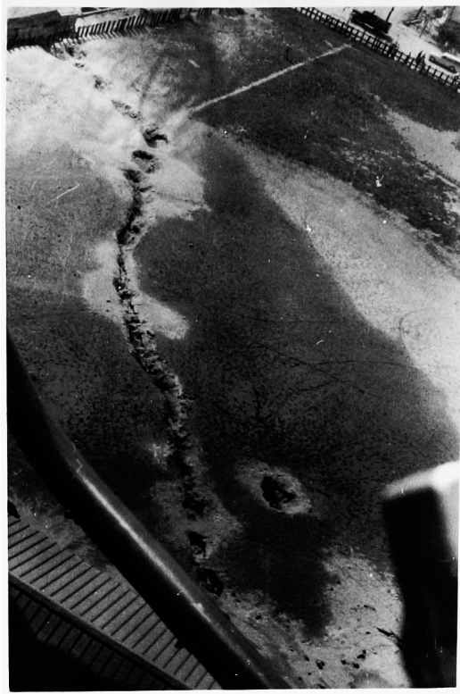
Fig.5 Ejecting holes in a row on the liquefied ground in the Niigata earthquake, June 16, 1964.
