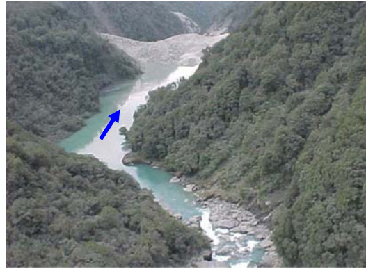
(b) October 6 th 1999: aerial view looking down the Poerua River at lake building up behind landslide debris (from left) building up in the river bed.
