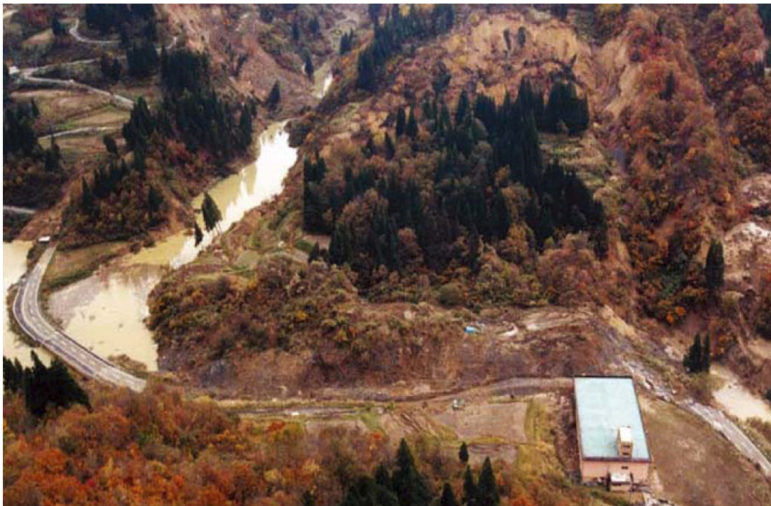
Front view of the Higashi-Takezawa Landslide
