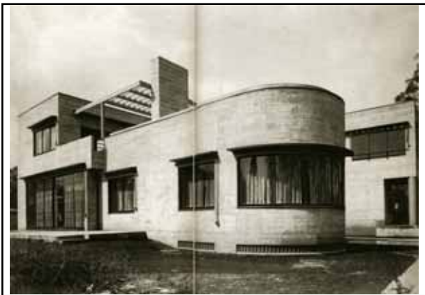
South facade (south-east view)
