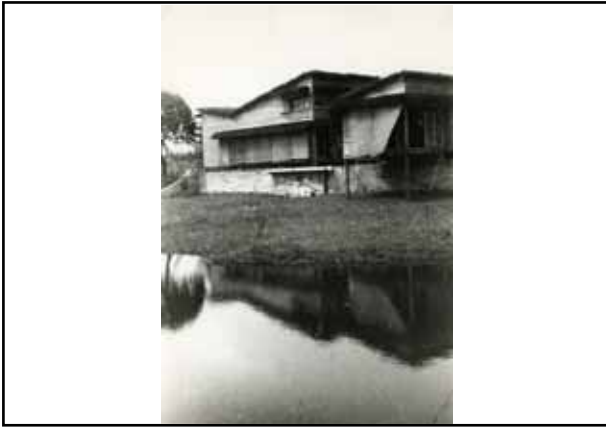
South-east view (with sudare blinds) with pond in the foreground
