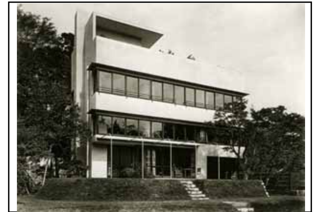
South facade with stairs leading to garden
