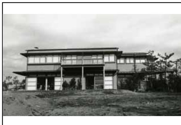
South facade with garden
