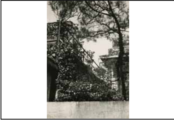
Roof garden handrail (view from garden)
