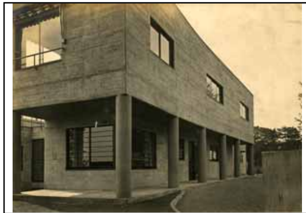
North facade (north-east view)
