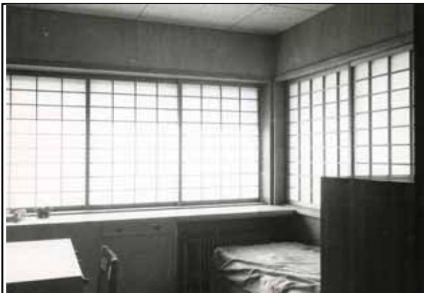
Bedroom windows with shoji (paper screens, 2F)
