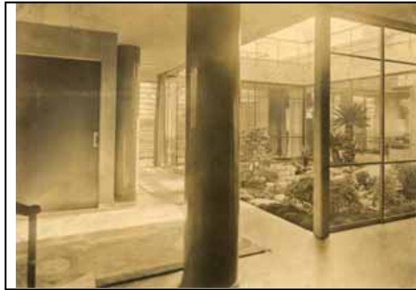
View of patio from living room (1F)
