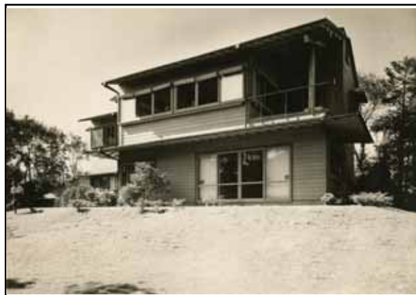
South facade with garden
