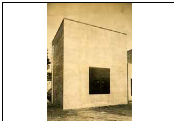
Kura with fireproof door
