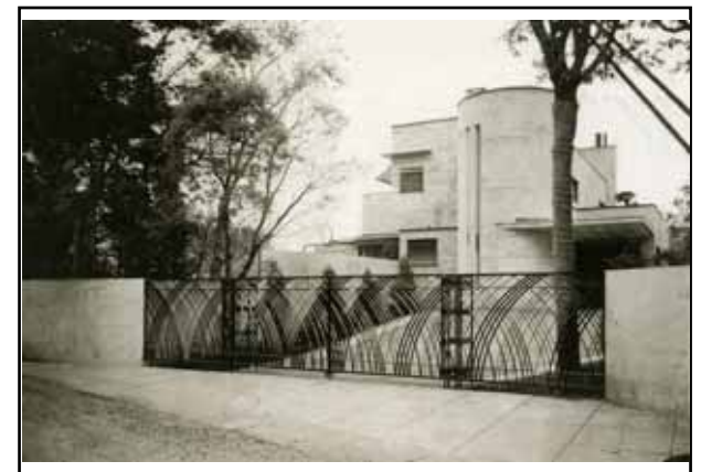
Approach with entrance gate (east)
