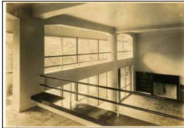
Mezzanine with windows opening onto the garden and living room fireplace below (2F)
