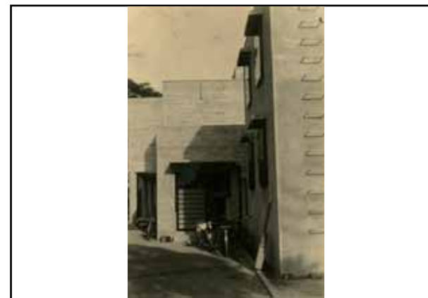
Kura with fireproof windows (right view)
