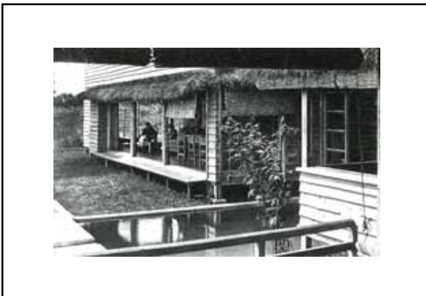
View of living room across from bedroom
