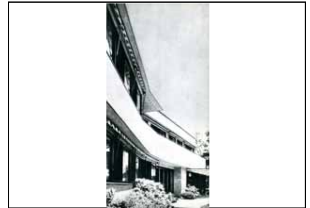
South facade (south-west view)
