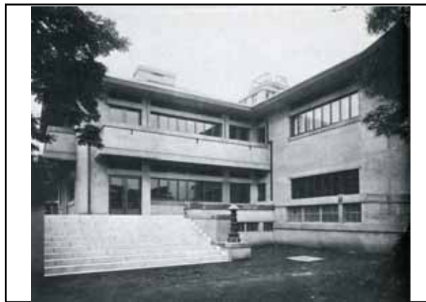
Close-up of rear stairs leading to terrace (south-east)
