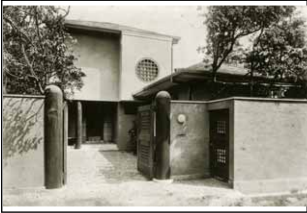
Street approach with front gate (west)
