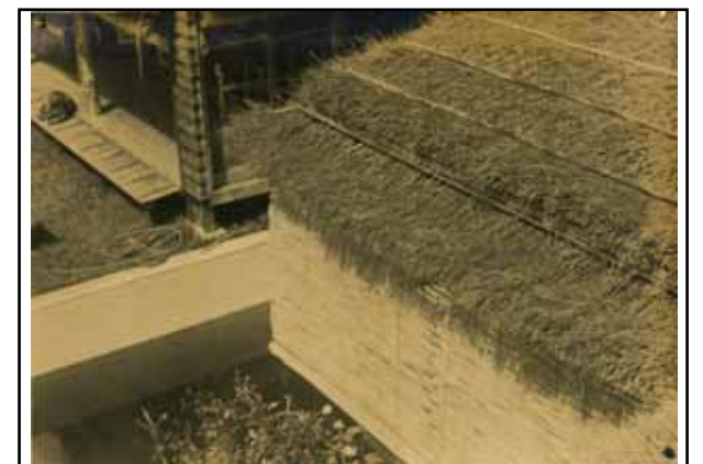
Thatched roof (larch)
