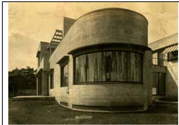
East facade (left part)
