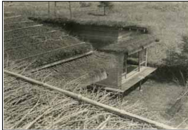
Thatched roof (larch)
