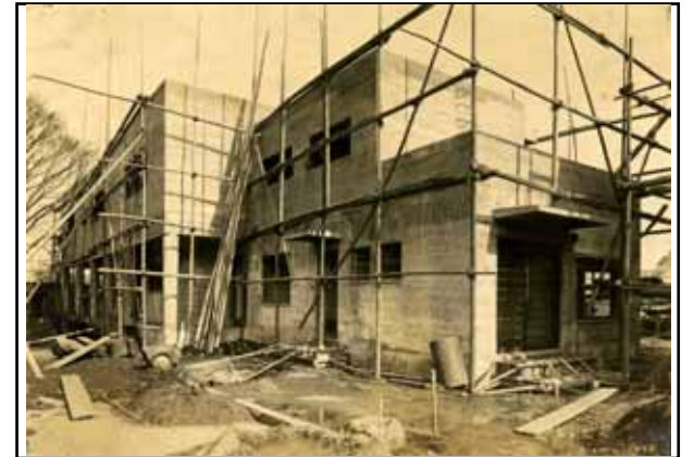
North facade (north west view)
