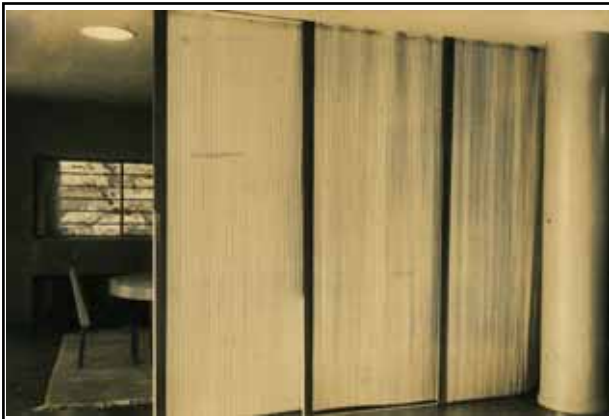
Sliding screens between dining room and living room (1F)
