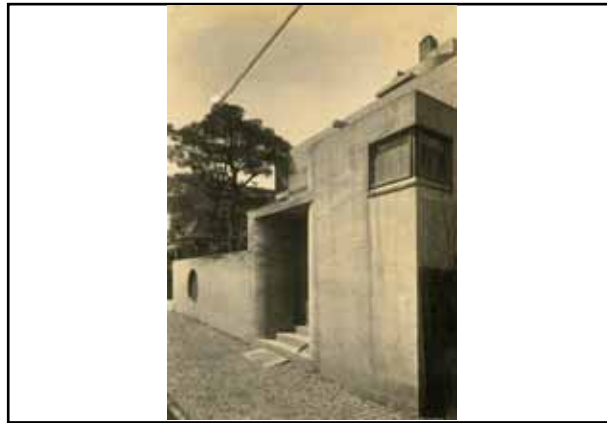
Street approach from north-east side
