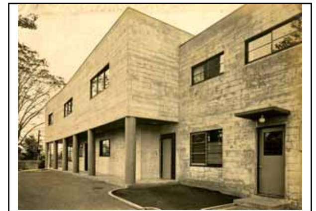
North facade (north-west view)
