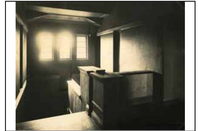
Staircase and landing (2F)
