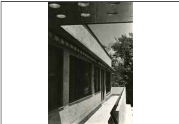
Windows and balcony
