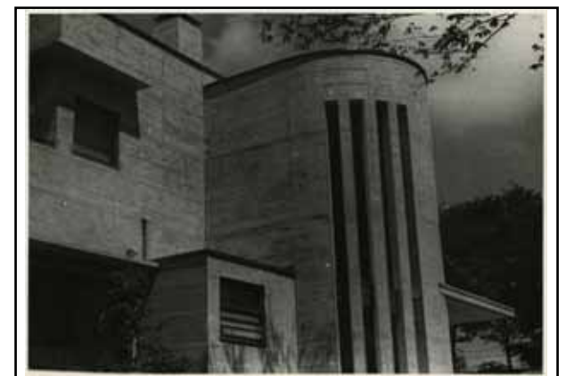
Staircase (east facade)
