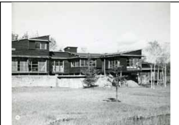
Karuizawa house after larch twigs have been removed from roof (south)
