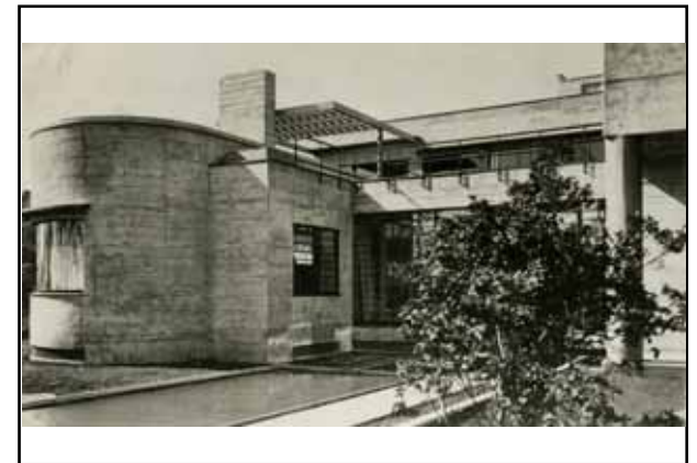
East facade with patio and pool
