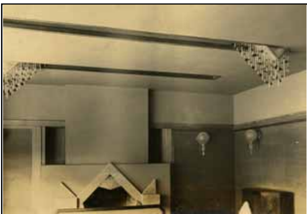
Reception room ceiling (1F)
