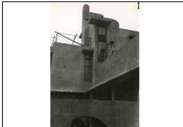
House under construction (view from street)
