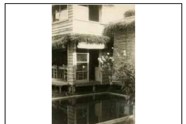
Pool, living room (1F) and studio above (2F)
