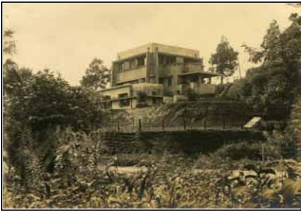
The house in its surroundings (south-east)
