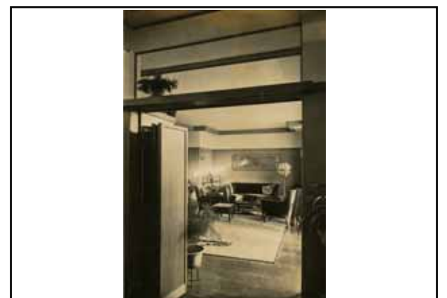
Living room seen from entrance hall (1F)
