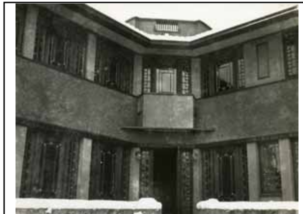
Close-up view of main entrance (south)
