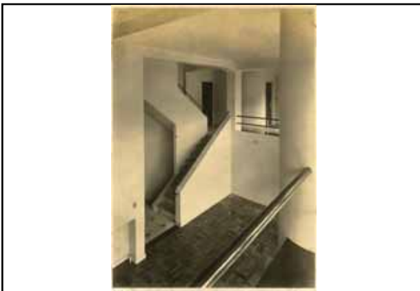
Living room with staircase seen from mezzanine (1F)
