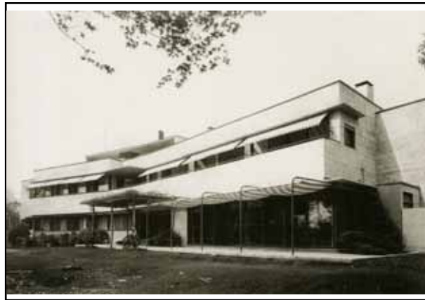
South facade (south-east view)
