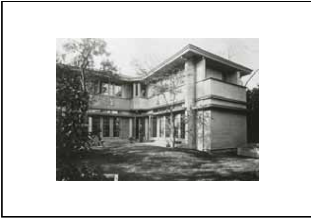
Front facade with corner entrance (south-east)
